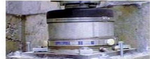
The close-up view of one of the Emery Winslow Model 136, 75,000-pound hydrostatic load cells used in the Bocker Grain installation.
