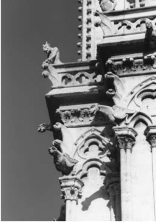
2. Chimeras on the western corner buttresses of the south tower, Notre-Dame, Paris (nos. 22 and 24), January 2000. (Photo: Stuart Michaels.)
