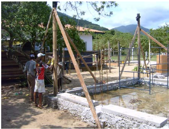
Figure 6.38. Placement of the bamboo columns. 2006.
