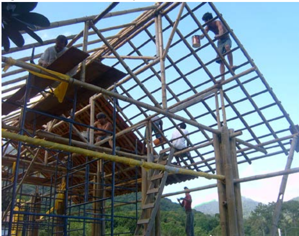
Figure 6.44. Varnishing of the bamboo. 2006
