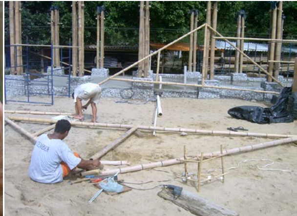
Figure 6.41. Scale model to help prefabrication of a module. 2006
