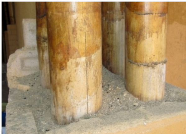
Figure 6.64. Bamboo poles protected by square brickwork made of adobe and filled with beach sand. 2017.
