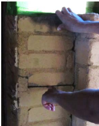
Figure 6.63. Detached bricks. 2017.
