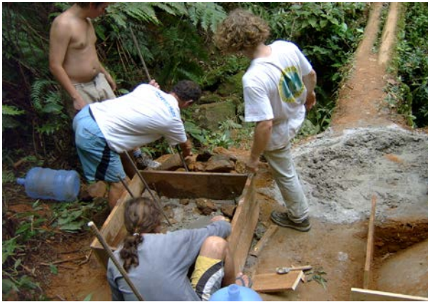
Figure 6.5. Concrete foundation for the bridge. 2004.
