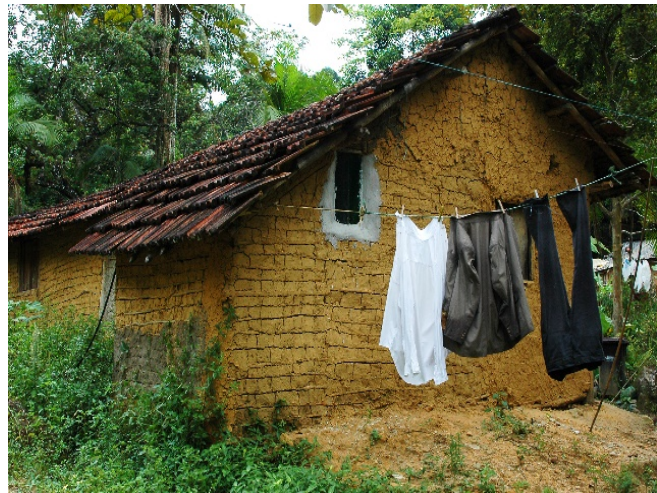
Figure 2.17. Wattle and daub house in Camburi, Brazil. 2006.
