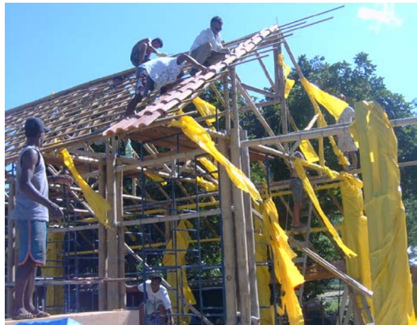
Figure 6.45. Placement of the roof tiles. 2006.
