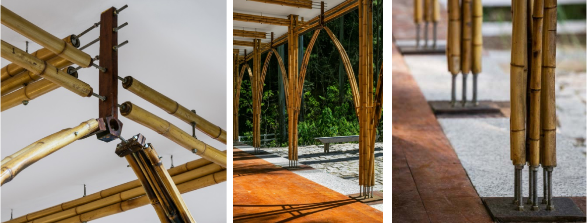
Figure 3.50. Violin connection and column connection. 2016. Copyright Nelson Kon.
