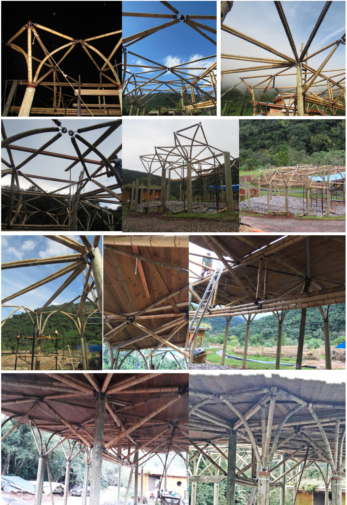
Figure 6.94. Construction process of the bamboo canopy, 2019.
