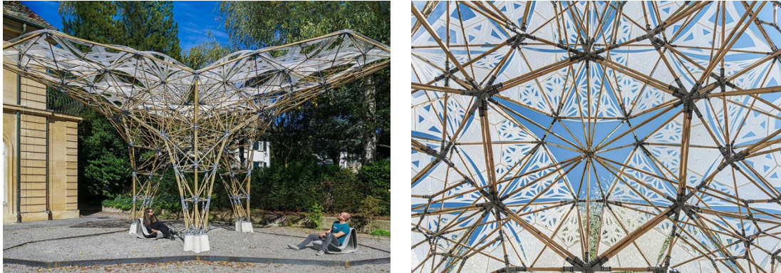
Figure 3.72. 3D printed joints. Retrieved on 06/02/2021 from https://www.designboom.com/architecture/eth-zurich-digital-fabrication-bamboo-pavilion . Copyright ETH Zurich / Marirena Kladeftira.
