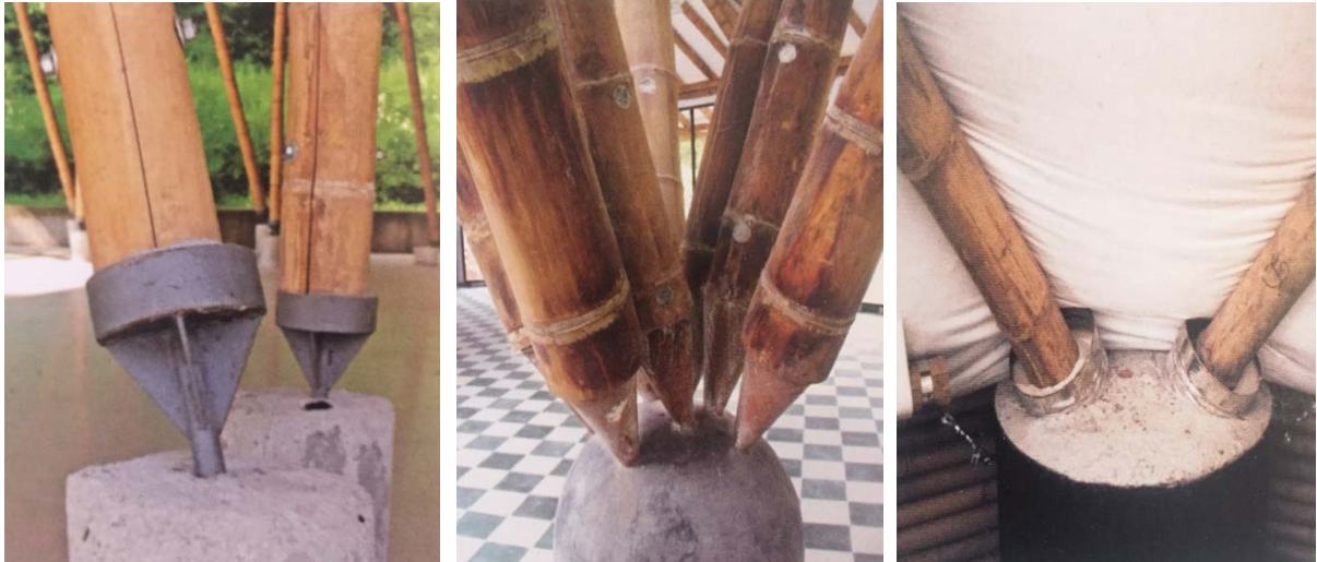
Figure 3.23. Potential solutions for bamboo foundations. Retrieved from Building with bamboo (p. 48,49) by G. Minke. 2012. Copyright Birkhauser.
