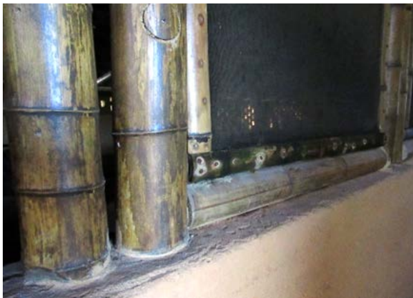
Figure 6.66. Darkening of bamboo poles. 2017.
