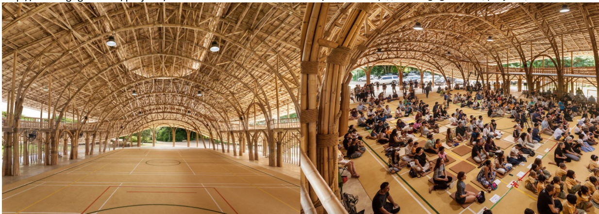
Figure 2.13. Sports hall Panyaden Int. School, Thailand. Retrieved from Chiangmai Life Construction website. 2019. https://www.bamboo-earth-architecture-construction.com/portfolio . Copyright CLC.
