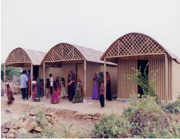
Figure 4.9. Paper Log Houses in India designed by Shigeru Ban. 2001. Retrieved on 26 February 2021 from www.archdaily.com/489255/the-humanitarian-works-of-shigeru-ban . Copyright Kartikeya Shodhan.
