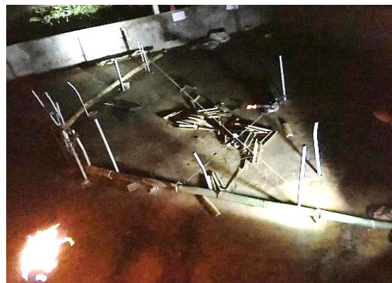
Figure 3.76. Securing the curvature with a rope. 2018.
