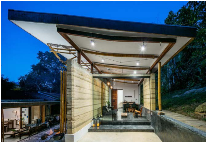
Figure 6.88. Inverted trusses. 2018. Copyright Nelson Kon.
