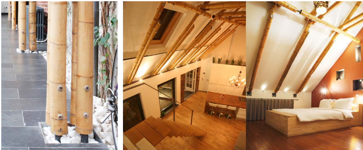
Figure 3.48. Column and ring beam connections in the bamboo house in Ghent. 2011.
