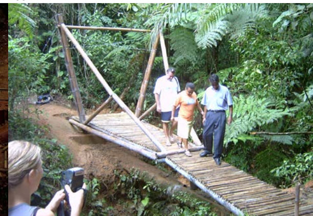
Figure 6.10. Completed bamboo bridge. 2005
