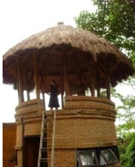
Figure 6.25. Completion of the bamboo canopy. 2006.
