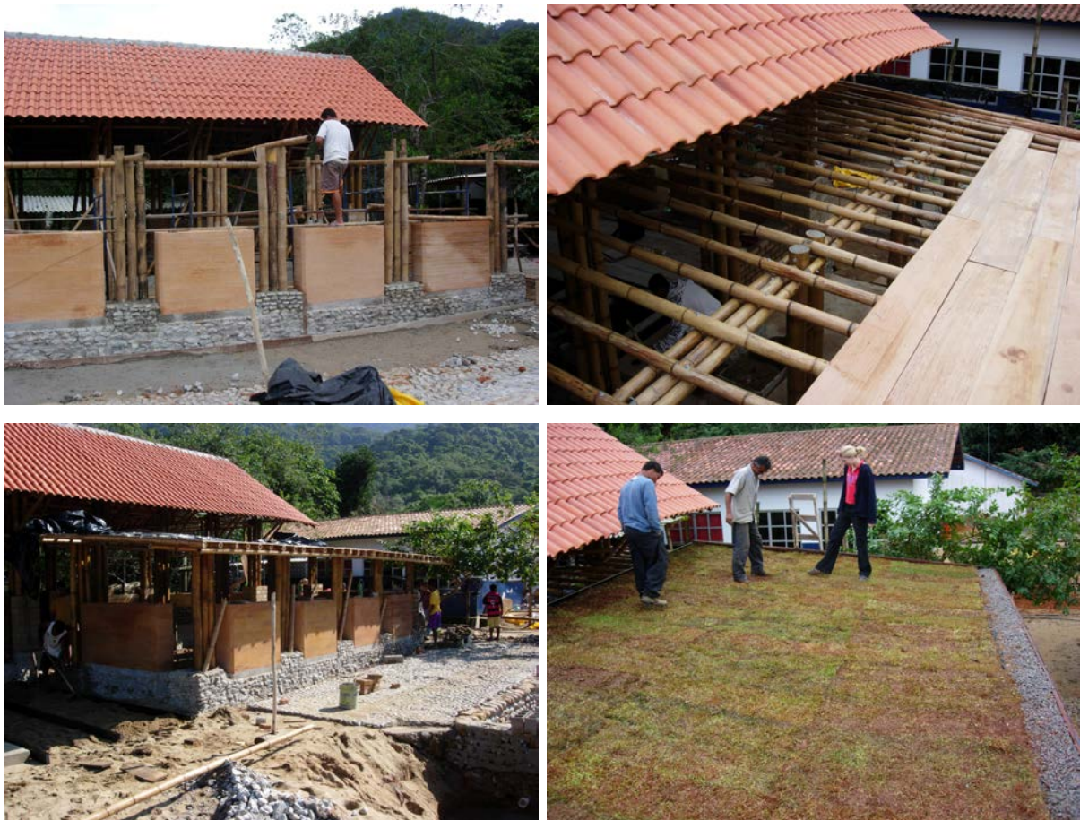
Figure 6.49. Construction of the green roof for the preschool. 2006.
