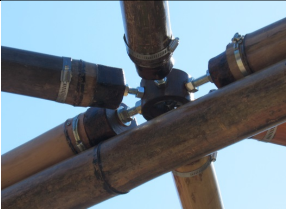
Figure 3.66. Central joint connecting the A modules. 2019.
