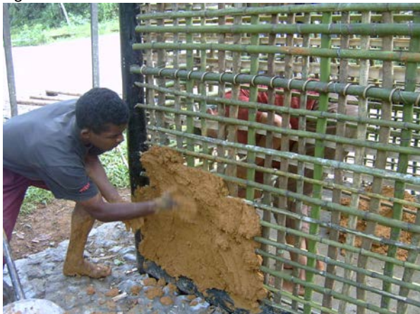
Figure 6.21. Wattle and daub technique. 2005.
