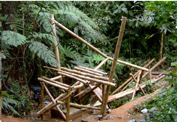
Figure 6.6. Scaffolding in Bambusa Vulgaris . 2004.
