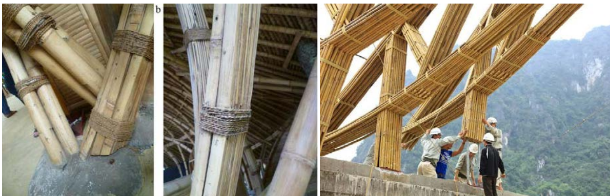
Figure 3.6. Bending and bundling of split bamboo. Retrieved from The potential of bamboo as building material in organic shaped buildings (p. 37) by E.A. Nurdiah. 2016. Procedia.
