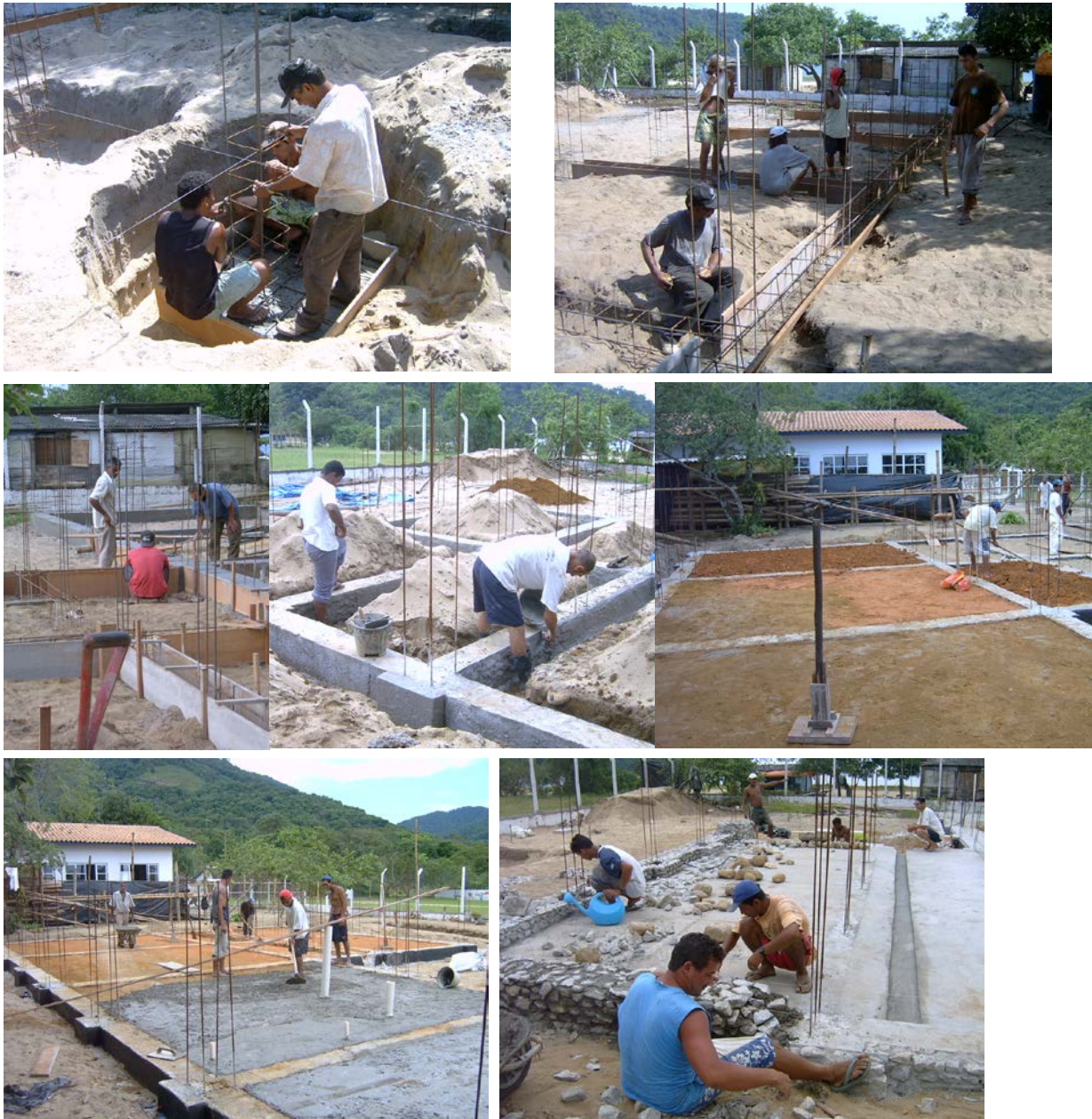
Figure 6.37. Process of the foundation. 2006.
