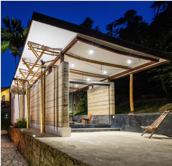
Figure 6.86. Interior and exterior trusses. 2018. Copyright Nelson Kon.
