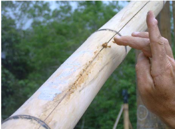
Figure 6.40. Mixture of sawdust and glue to close off cracks. 2006
