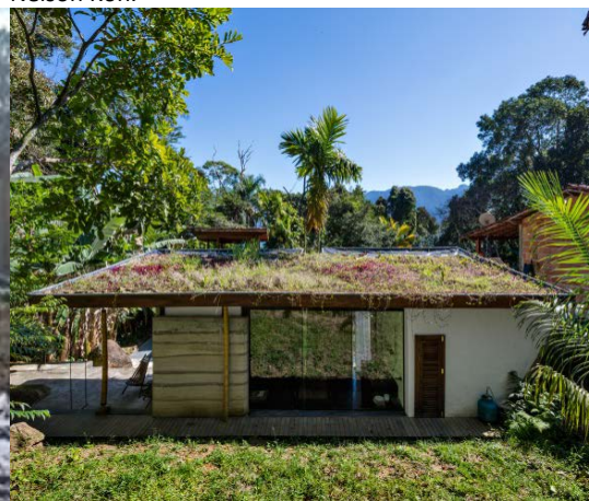
Figure 6.91. Green roof. 2018. Copyright Nelson Kon.
