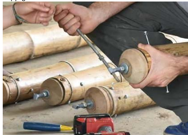
Figure 3.28. Wooden connector piece by Y. Barnet & F. Jabrane of Forestbambú Perú. 2019. Retrieved from https://www.forestbambu.com/noticias (05/04/2020). Copyright Forest Bambu.
