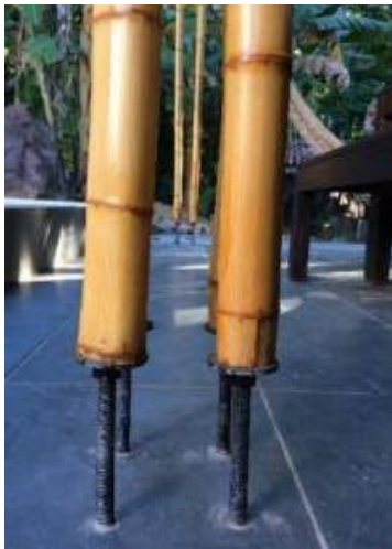
Figure 6.69. Column base supporting on wire rods. 2016.
