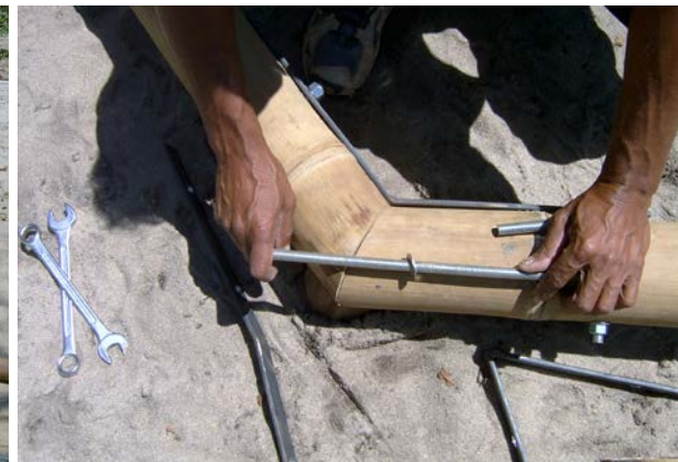
Figure 6.8. Bamboo connection with an outer steel plate. 2004.
