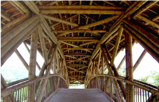
Figure 2.5. Bamboo bridge Santa Fé, Colombia. Retrieved from Building with Bamboo (p.151) by Gernot Minke, 2012. Basel, Birkhäuser. Copyright Birkhäuser.
