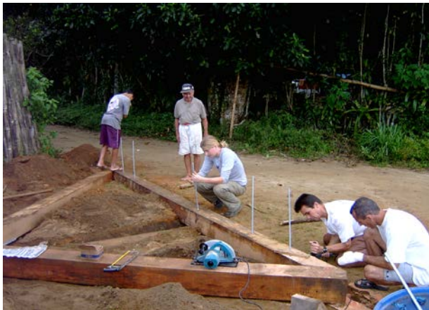
Figure 6.14. Hard wooden foundation. 2005.
