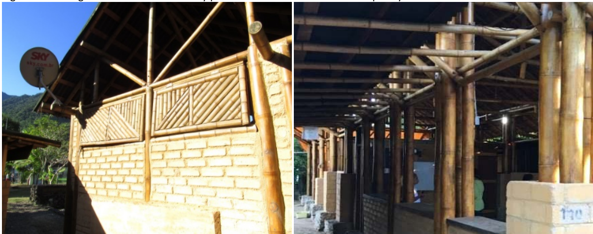
Figure 6.57. Exposed vertical bamboo members in good condition. 2017.
