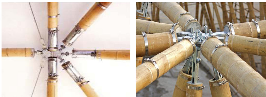
Figure 3.31. Internal metal connector pieces (Group 2). Retrieved from Design with nature (p.81,82) by M. Heinsdorff. 2011. Copyright Hirmer Publishers.
