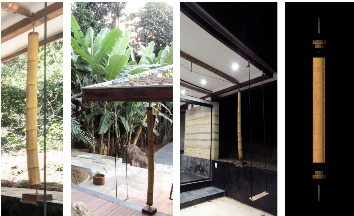
Figure 7.6. Single bamboo pole column used in the guesthouse in Brazil.
