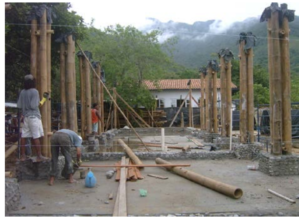
Figure 6.39. Plastic to cover the bamboo ends. 2006.
