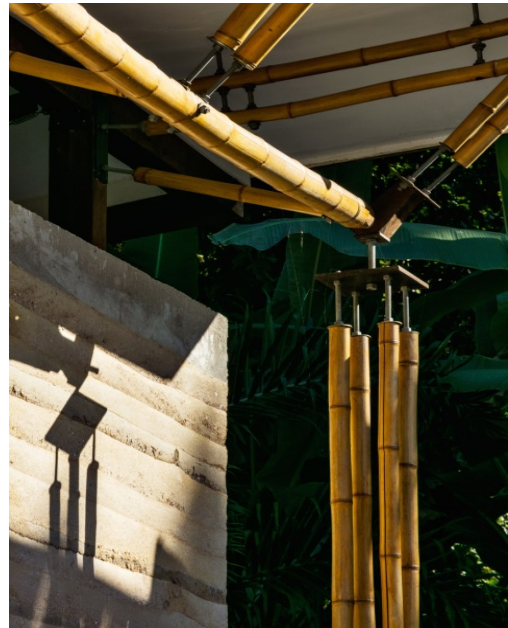
Figure 6.87. Detail of exterior truss and column. 2018. Copyright Nelson Kon.
