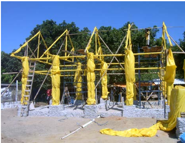
Figure 6.43. Process of the placement of the trusses. 2006.
