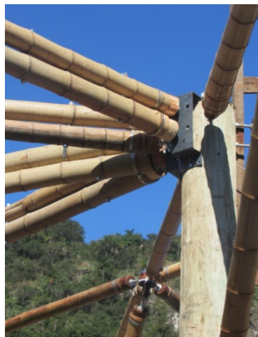
Figure 3.62. The connection of the beams to a eucalyptus column. 2019.
