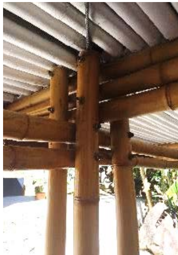
Figure 6.70. Detail of top of the column. 2016.
