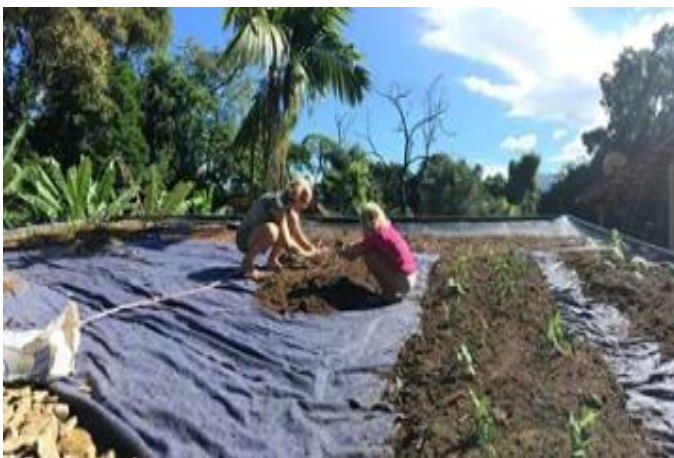
Figure 6.90. Earth layer for the green roof. 2018.
