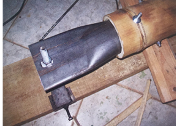
Figure 3.26. Connector piece by Vitor Marcal. Retrieved from Building with bamboo (p. 45) by G. Minke. 2012. Copyright Birkhauser.
