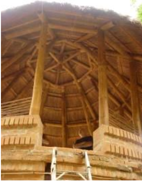
Figure 6.24. Kingpost bamboo structure. 2006.
