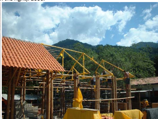
Figure 6.48. Completion of the main roof. 2006.
