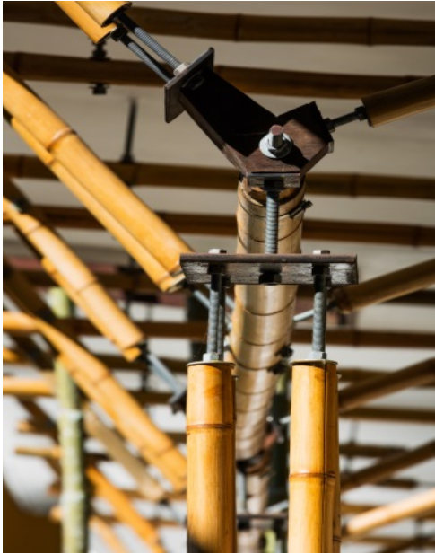
Figure 6.84. Detail of the bird joint. 2018. Figure 6.85. Bamboo column. 2018. Copyright Nelson Kon. Copyright Nelson Kon.
