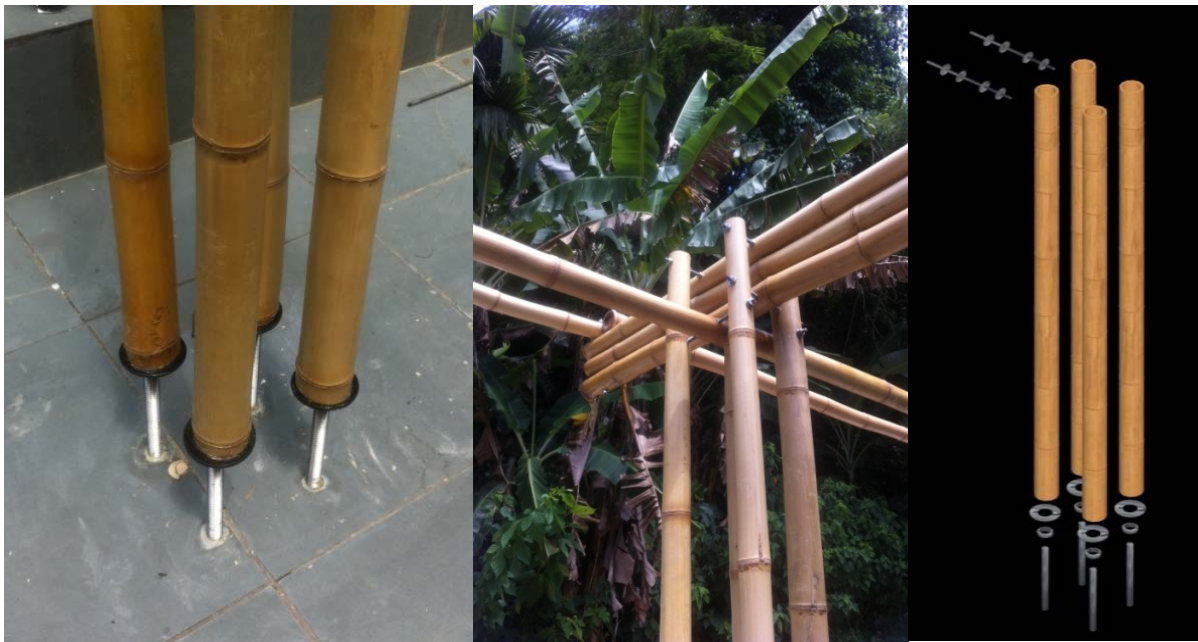
Figure 7.12. Four small diameter bamboos that form a coherent column in the veranda, Brazil.
