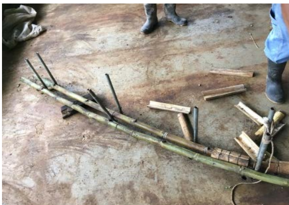
Figure 3.75. Two bamboo poles form one arch. 2018.
