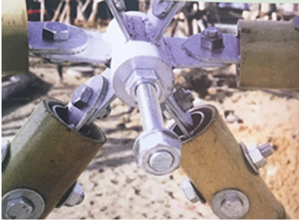
Figure 3.25. Connector piece by Hamura Shoei Yoh. Retrieved from Building with bamboo (p. 45) by G. Minke. 2012. Copyright Birkhauser.
