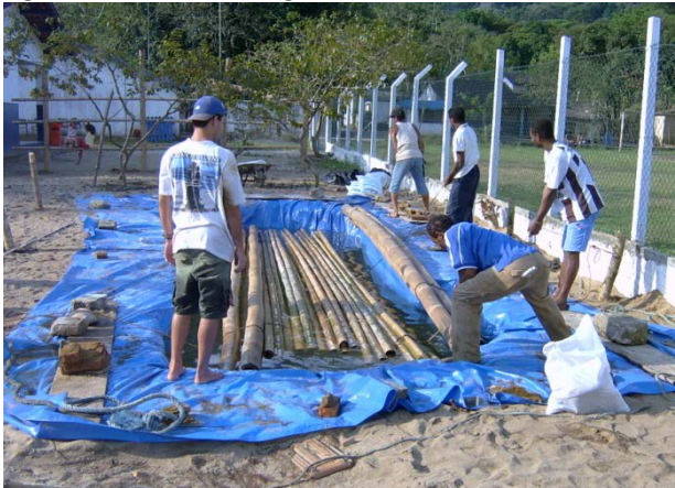
Figure 6.35. The borax treatment by diffusion. 2005.
