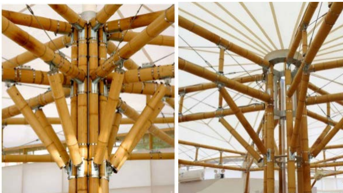
Figure 3.36. External metal connector pieces (Group 3). Retrieved from Design with nature. The bamboo architecture (p.47,55) by M. Heinsdorff. 2011. Copyright Hirmer Publishers.
