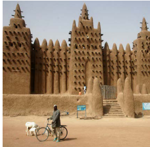
Figure 4.6. Mosque of Djenné. Radical Architecture Climate Change. Retrieved on 11 June 2019 from an online article by P. Harper. http://dezeen.com/2019/06/11/radical_architecture_climate_change-opinion-phineas-harper .
