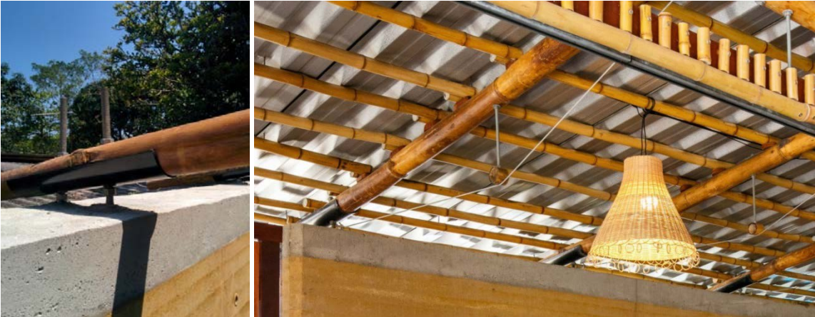
Figure 3.55. Inverted truss and half-tube connection. 2018. Copyright Nelson Kon.
