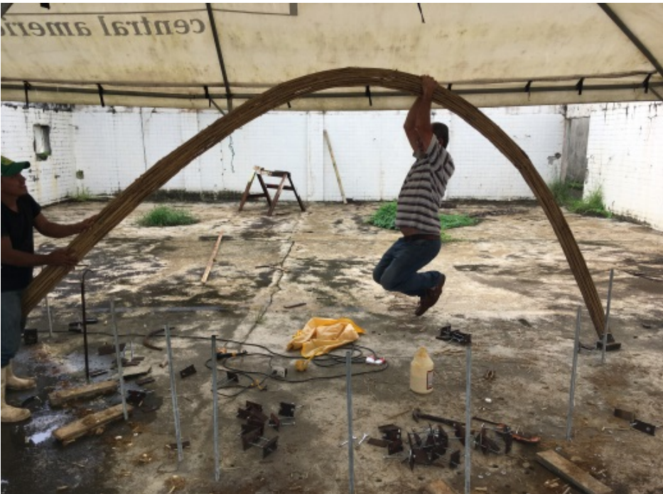
Figure 3.78. Process of the cold-bundling technique with glued bamboo strips. 2018.
