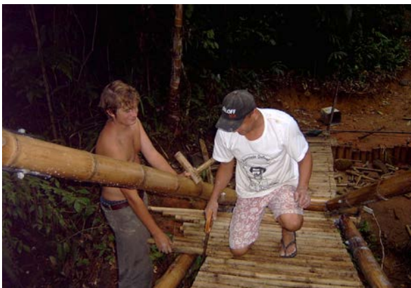
Figure 6.9. Making of bamboo walkway. 2004.
