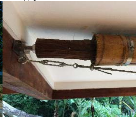
Figure 6.89. Wooden plug detail. 2018. Copyright Nelson Kon.
