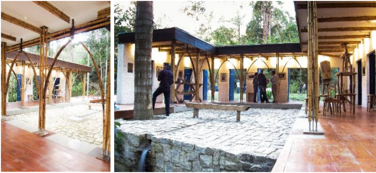
Figure 6.82. Completed art gallery. 2016.
