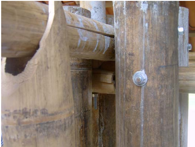
Figure 6.46. Joint failure (on the left) and the repair thereof (on the right). 2006.
