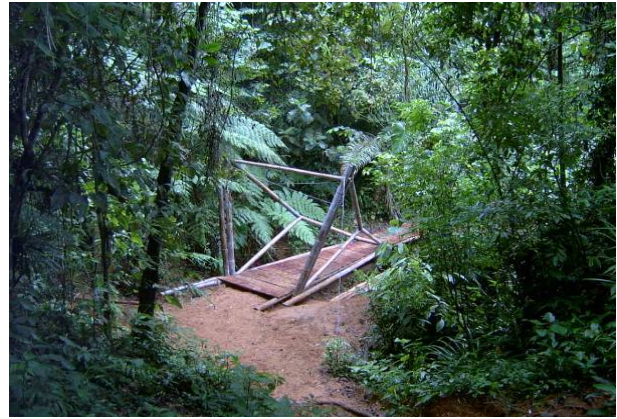
Figure 6.12. Bamboo bridge with hard wooden timber walkway. 2005.
