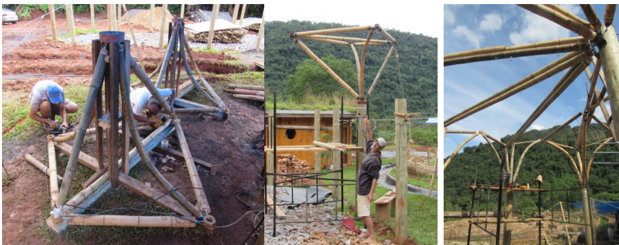
Figure 3.63. Both modules when finished. 2019.
