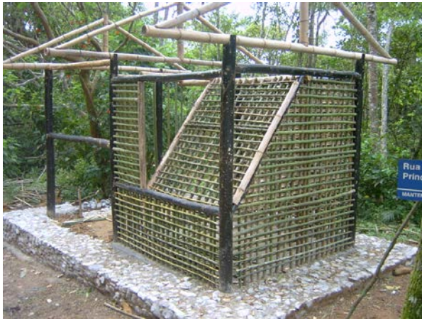
Figure 6.19. Bamboo frame for wattle & daub. 2005.
