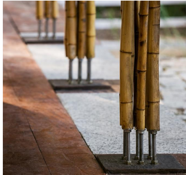
Figure 6.79. Detail of the foot of a bamboo column. 2016.
