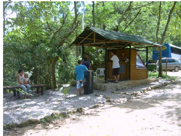
Figure 6.22. Completed information booth. 2005.
