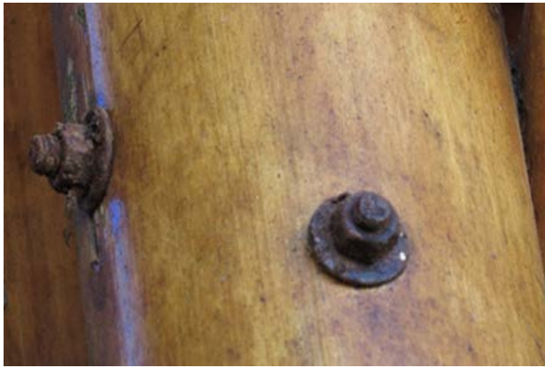
Figure 6.65. Corrosion of galvanized wire rods, hex nuts and washers. 2017.
