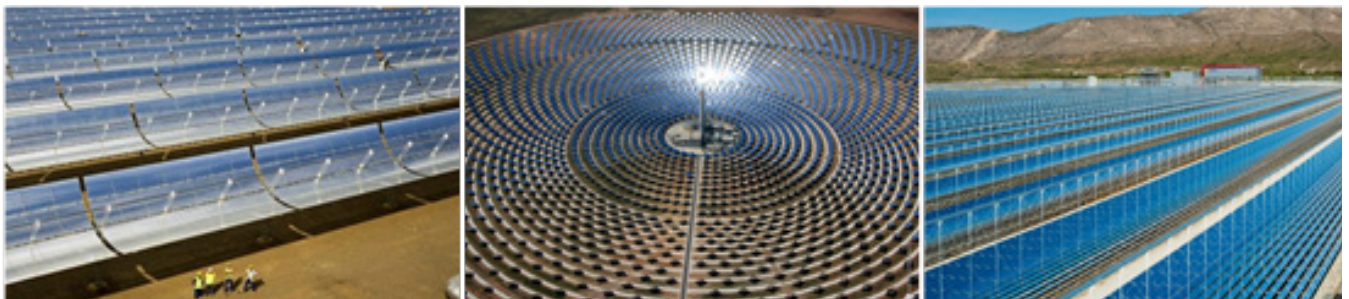
Figure 1: Considered CSP-Technologies (from left to right): Parabolic Trough (PT), Solar Tower (ST) and Linear Fresnel (LF)
