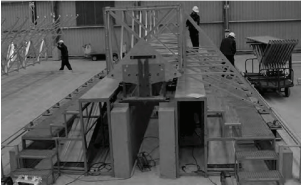
Figure 8: Exemplary assembly rig for a SCE (here Flagsol ) [6]
