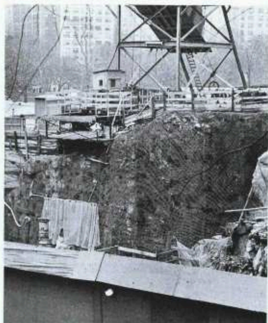
Construction, Central Park, New York City.
