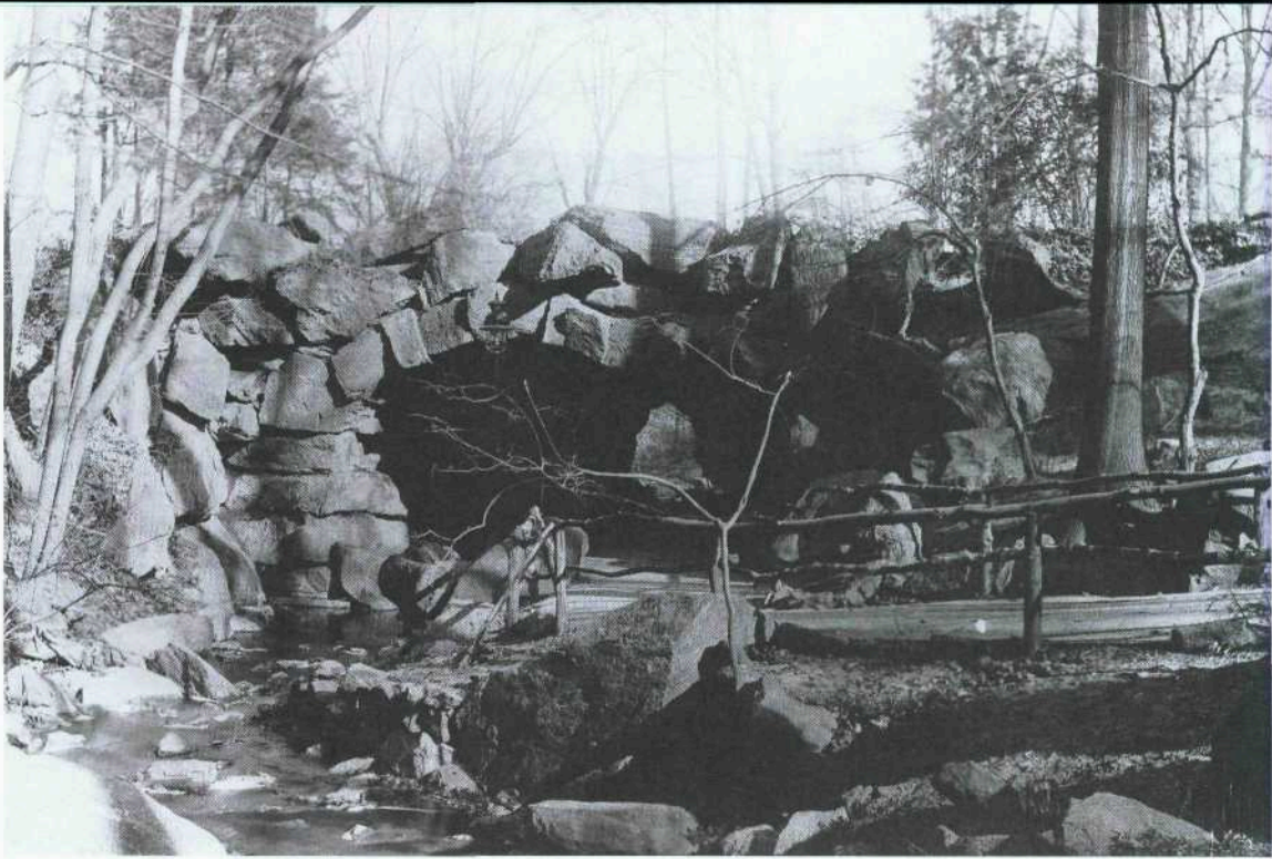
One of the many Central Park bridges, before 1900.
