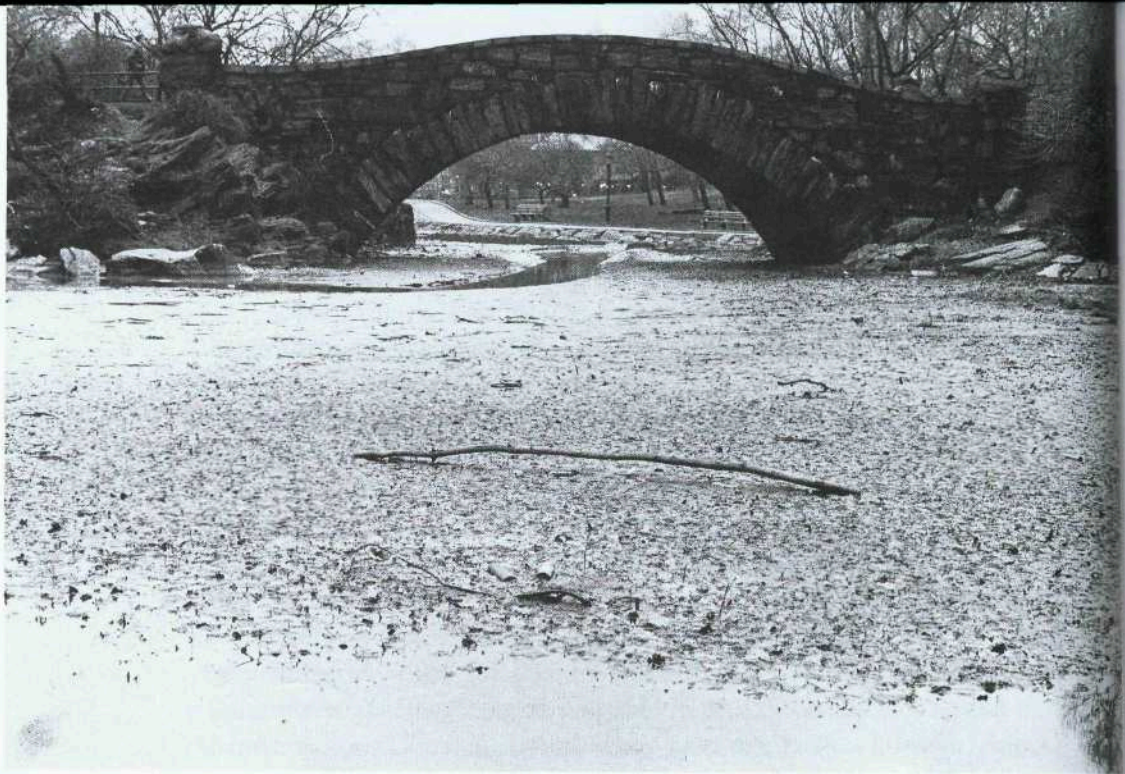
Gaptow Bridge with mud slough, 1972.
