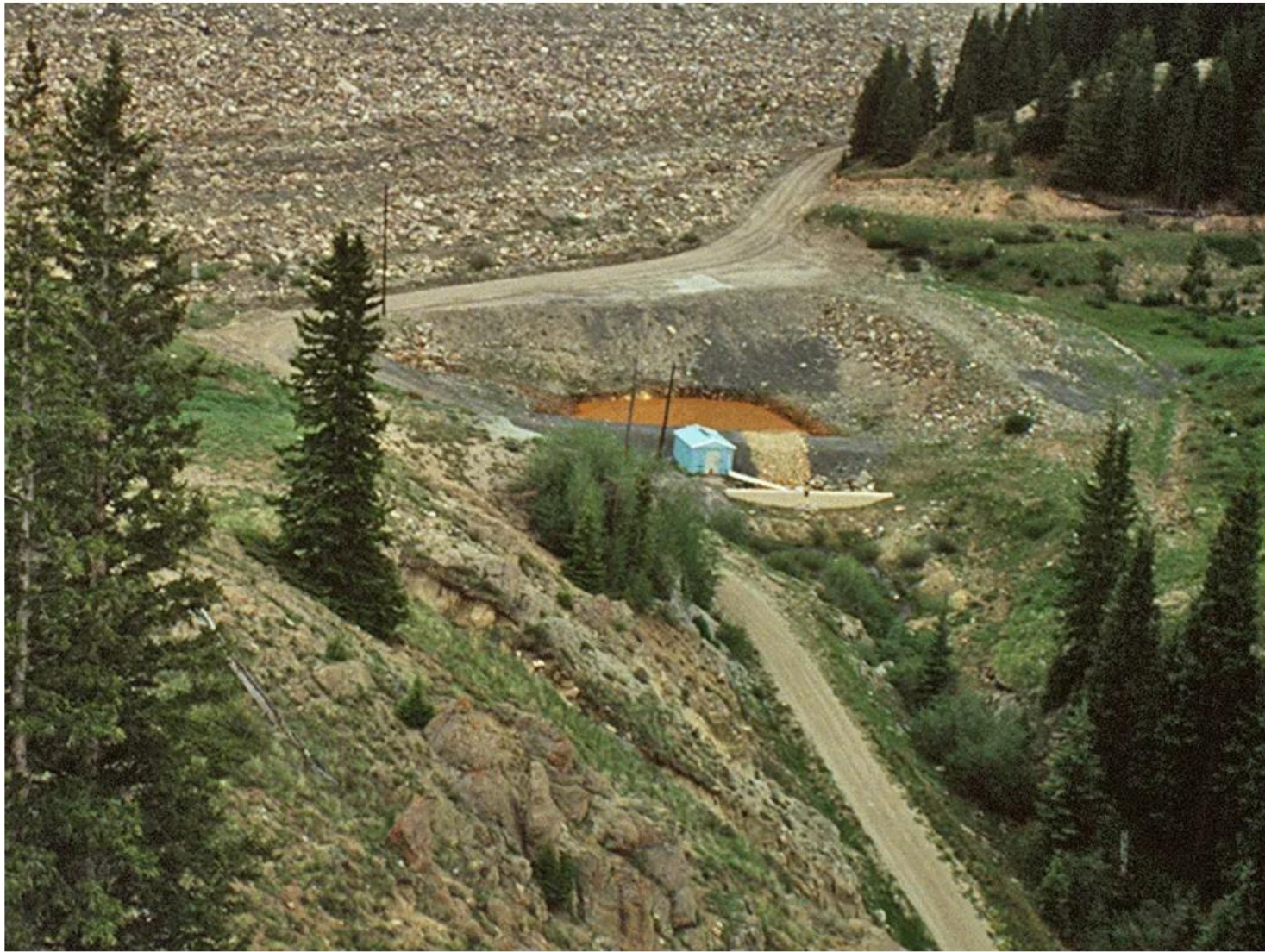
Mines often produce waste, or tailings, that contains chemicals, minerals, and heavy metals and gets stored in ponds like this one in Lake County,
