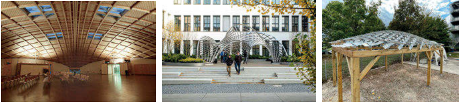
Fig. 1: Two gridshells with high node congruence and straight development: the Polydome at EPFL (left) and the Inside/Out Pavilion at TU Munich (middle) and the pseudo-geodesic gridshell (right).
