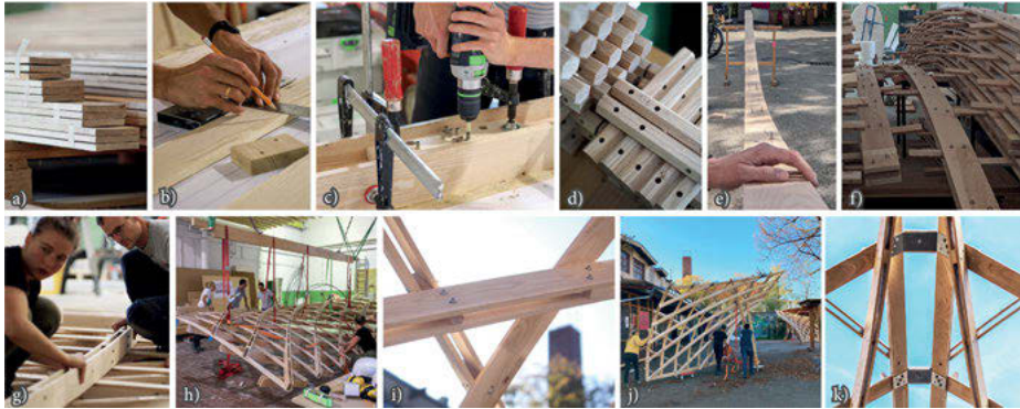
Fig. 7: Top Row: Prefabrication. 12 \times 100 mm planks (a) are marked (b), drilled (c), and coupled with 24 mm studs (d) into pre-bent (e) beams (f). This process embeds the geodesic curvature. Bottom Row: Assembly and Erection. The asymptotic beams and geodesic planks are interlaced into flat segments (g), and deformed into the doubly curved shape (h). The combination of asymptotic and geodesic planks (i) creates a stiff shell, that is transported (j) and assembled (k) on site.
