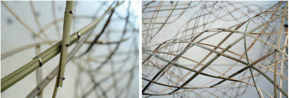
Fig. 7: Detail of the overlapping between bamboo slats (left); Connections occurring when cylinders start to shape nodes (right).
