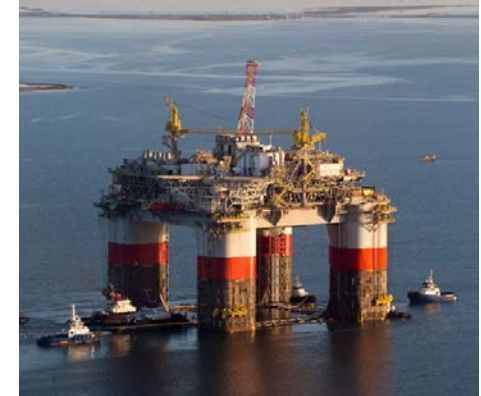
GoM – Chevron JSM - $7.5bn Installed 2014
