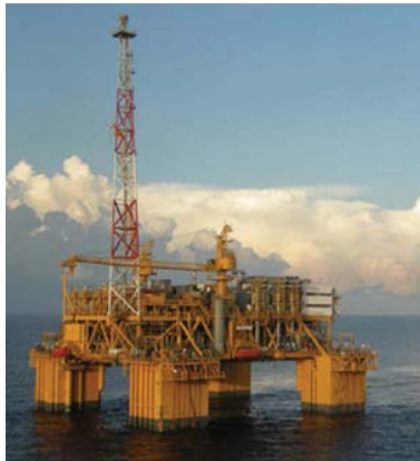
GoM – Anadarko I-Hub - $2bn Installed 2007
