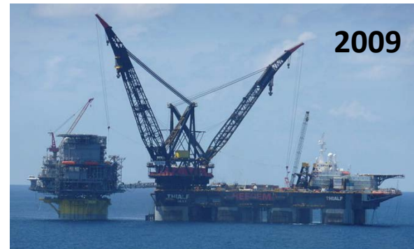
The Perdido spar is the deepest floating oil platform in the world at a water depth of about 8,000 ft. It was installed 200 miles from shore and is operated by Shell in the Gulf of Mexico.
