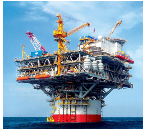
GoM – Chevron Tahiti - $2.7bn Installed 2009
