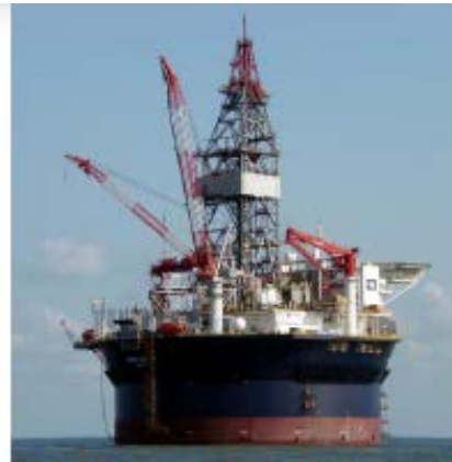
Sevan, MonoBR Circular FPSO (wet tree, worldwide)
