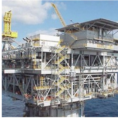
GoM – Exxon Hoover - $1.2bn Installed 2000
