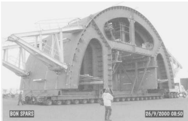
Figure 7.78 Rollout of Half-section (Technip Offshore)
