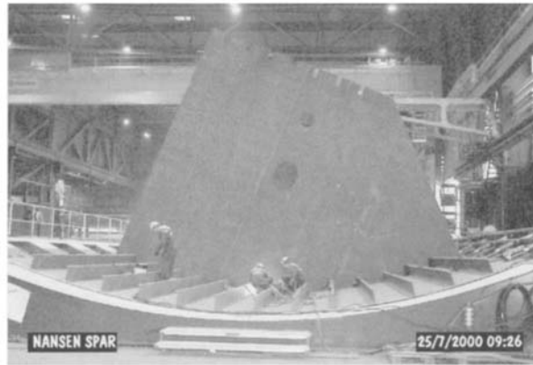
Figure 7.91 Forming the outer shell of spar platform, plating, stiffeners and bulkhead shown (Technip Offshore)
