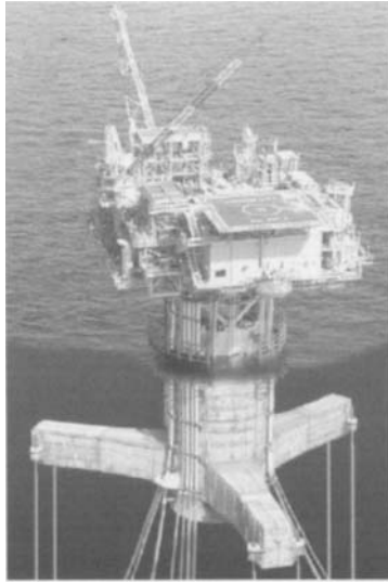
Figure 2.11 SeaStar MiniTLP for Typhoon Field (Reproduced courtesy of Atlantia Corporation)
