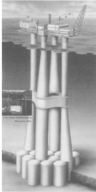
Figure 1.4 Troll A gas platform, world’s tallest concrete structure
