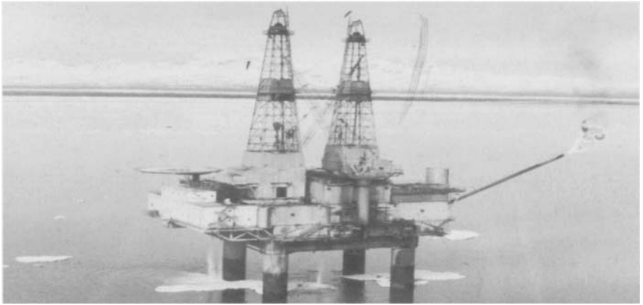
Figure 2.3 Tower type cook inlet platform
