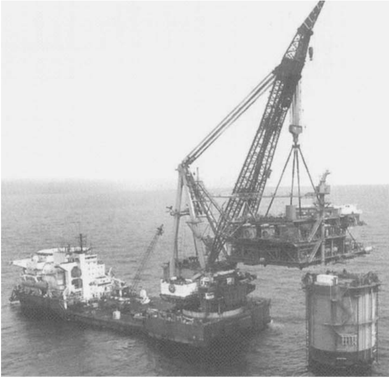
Figure 7.87 Derrick barge setting deck on spar platform (Technip Offshore)
