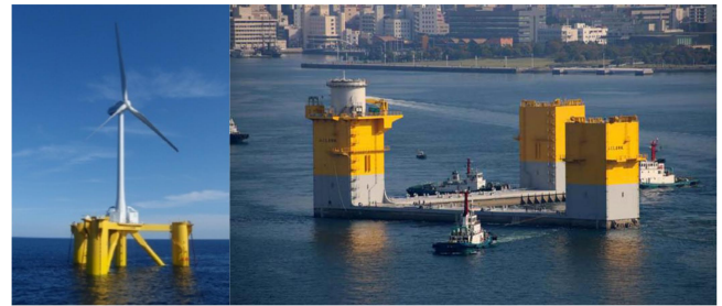
Fig. 1 Examples of FOWT with three columns in a triangular disposition: left, the Fukushima Mirai Wind Turbine; right, the Fukushima Shimpuu Wind Turbine
