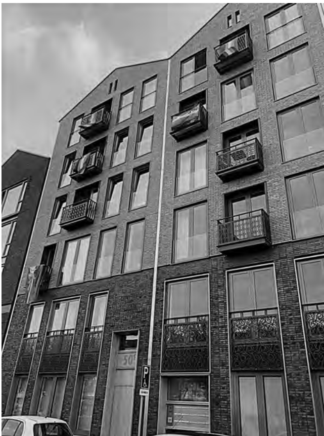
FIGURE 6.2 Rainbow flags at Roze Hallen housing project, Amsterdam Oud-West area. Source: Josée Rothuizen, 2018.
