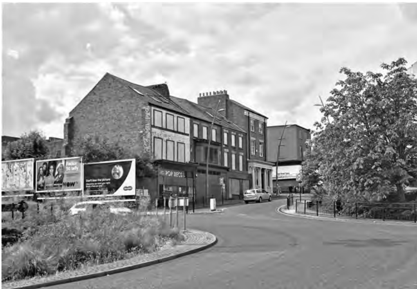
FIGURE 19.2 The first three buildings 170/5 High Street West Sunderland. Source: Loes Veldpaus, 2019.
