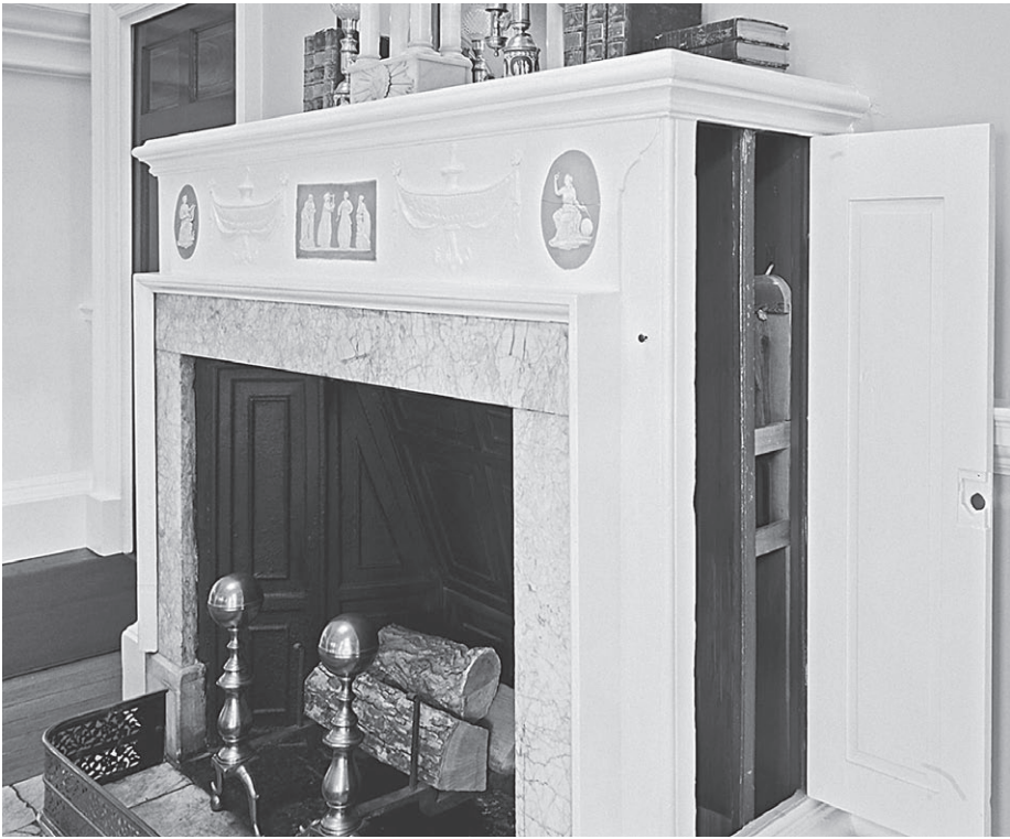
Fig. 3.6 Thomas Jefferson, Monticello, 1770–1809. Dumbwaiter built into dining room fireplace. Courtesy of Thomas Jefferson Foundation.
