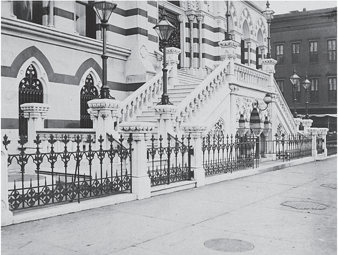
Fig. 6.3 P. B. Wight, National Academy of Design, New York, 1865. Entry staircase from the southwest corner of the building showing the newels of the stairway. National Academy of Design: Photographs of the New Building , with an introductory essay and description by P. B. Wight (New York: S. P. Avery, 1886). Courtesy of Metropolitan Museum of Art.
