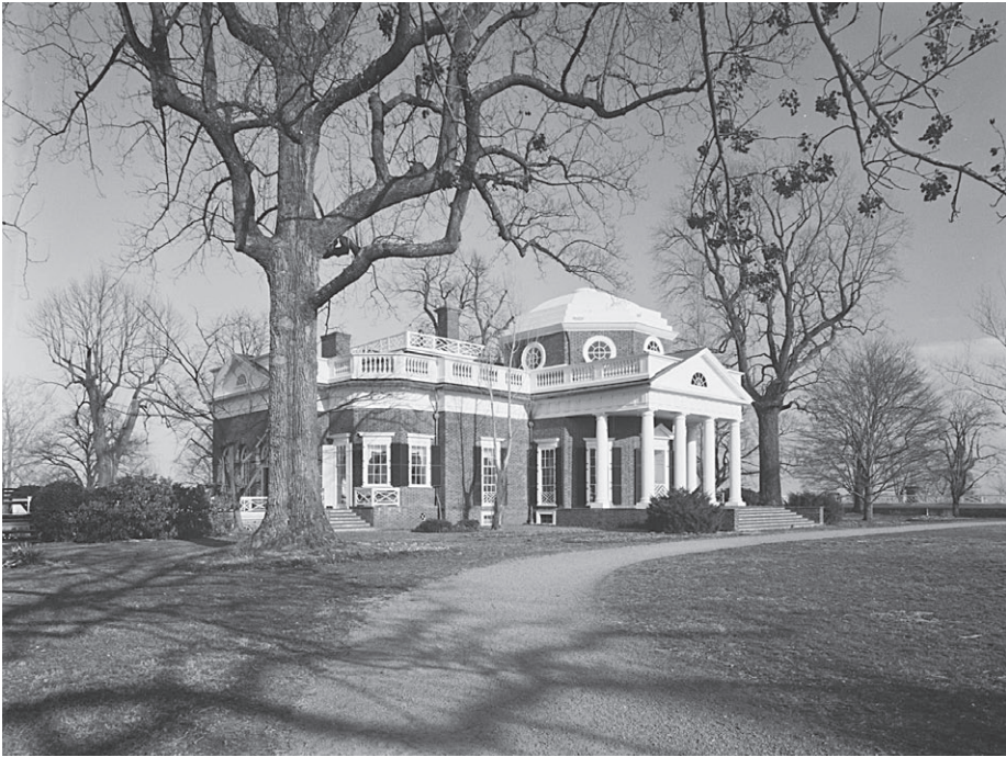
Fig. 3.4 Thomas Jefferson, Monticello, 1770–1809. West facade from the northwest. Historic American Buildings Survey, n.d. Library of Congress, Prints and Photographs Division.
