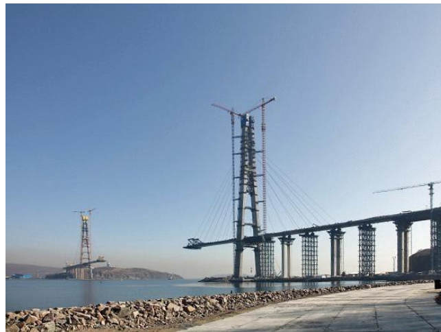
Bridge to Russky Island – Russia, 2012 Estaiada – Vão de 1104m
