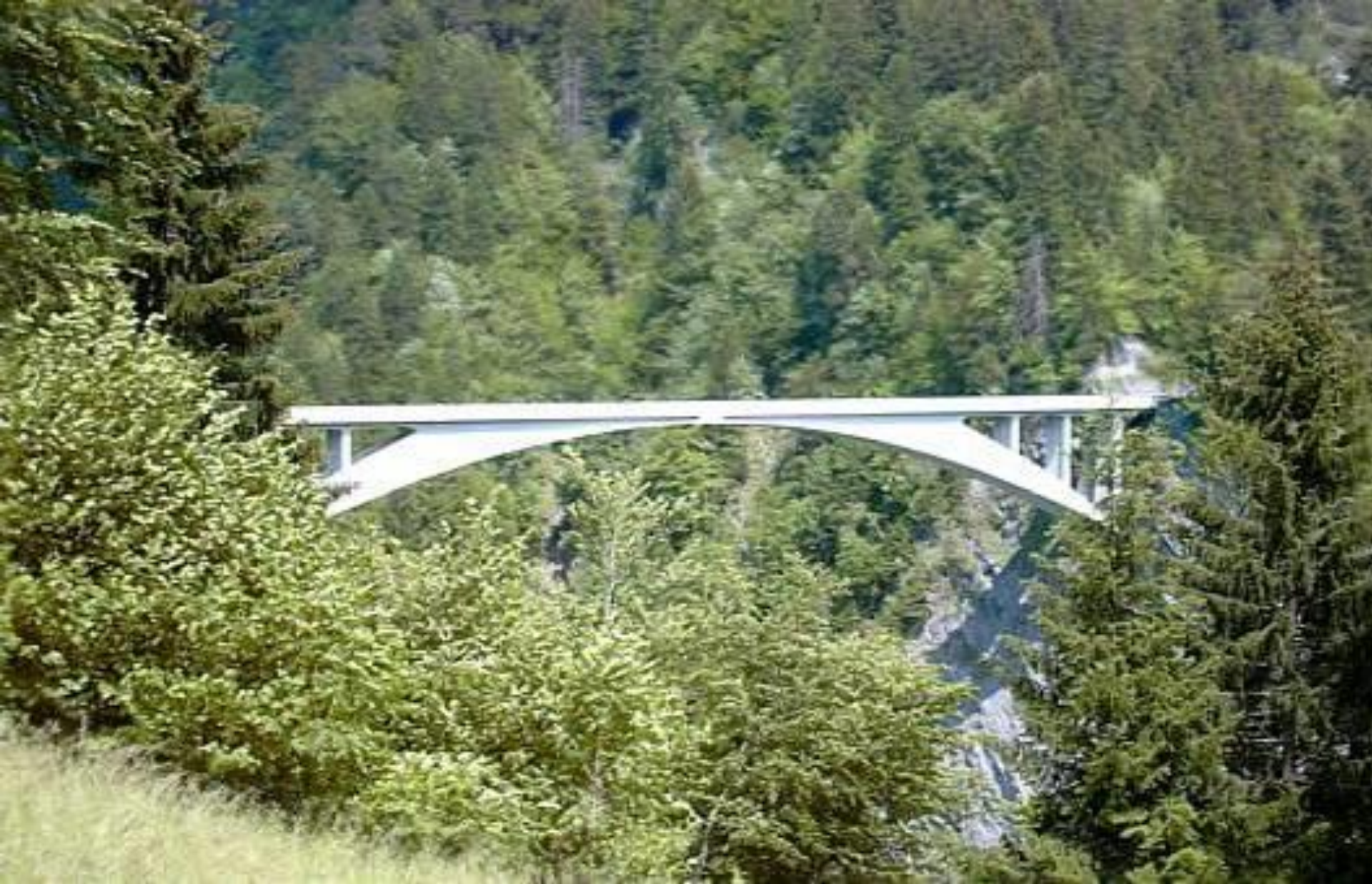
Ponte Salginatobel, Suíça Robert Maillart, 1929 (total length 133 metres, longest span 90 metres)
