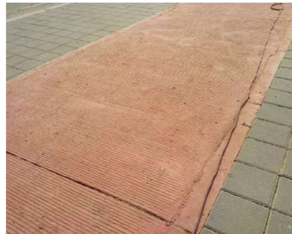
Fig. Broom finish on a cycle track in FC Road, Pune
