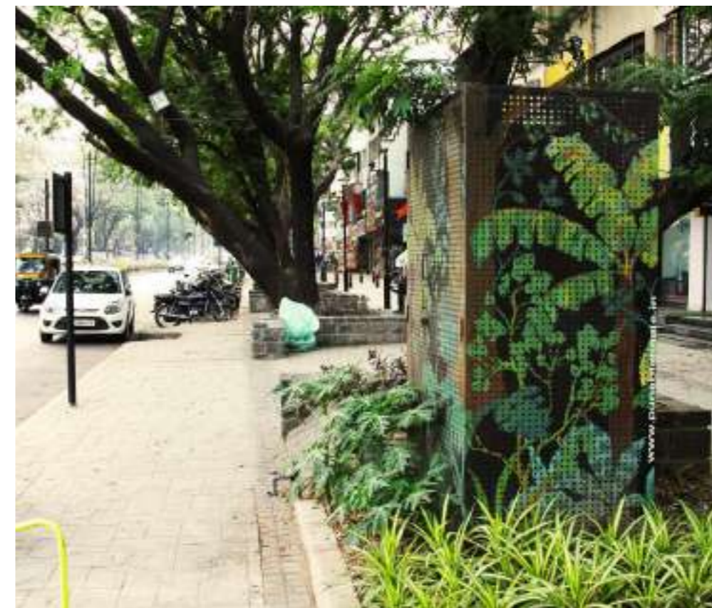
Fig. (above) Location of manholes in bulb-outs in JM Road, Pune
