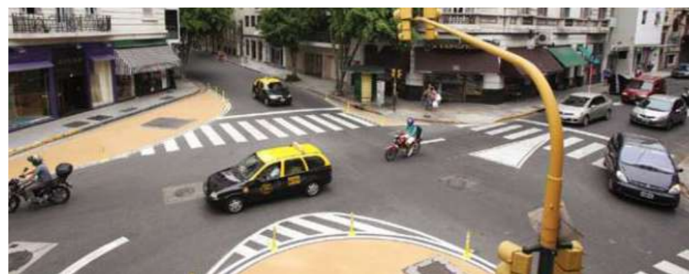
Fig. Testing out the redesign of a complex X-intersection in Buenos Aires with kerb extensions, refuges and a plaza.
