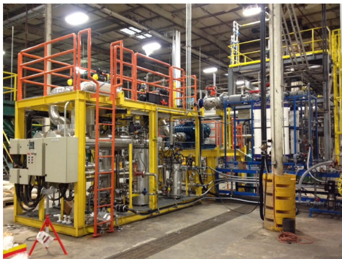
FIG. 7.4 25,000 L per day capacity AQUA SEP™ hybrid membrane distillation plant for sugar extraction and purification from MSW.
