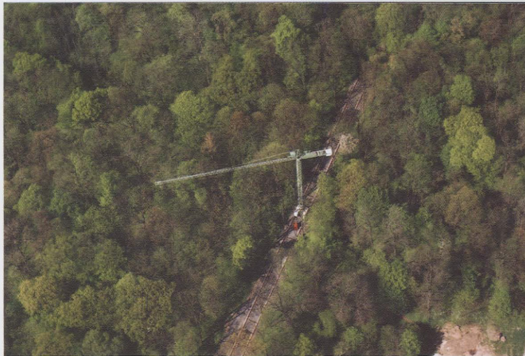
Figure 1 Aerial photo of crane and rail track. Courtesy UFZ Leipzig-Halle AG.
