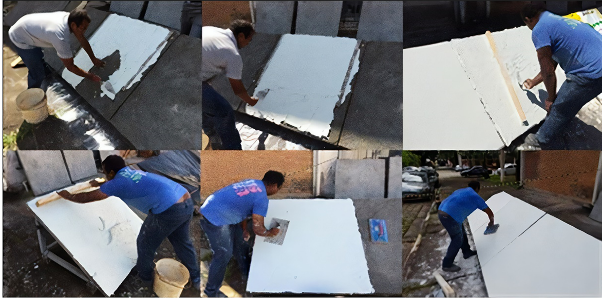
Fig. 5. Mortar application by mason in situ.
