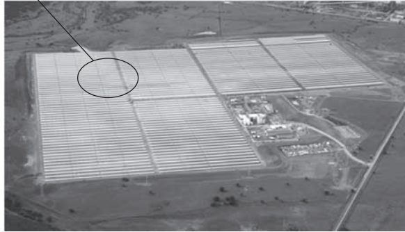
7.15 Parallel rows in a solar field with parabolic-trough collectors.
