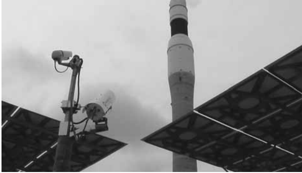
8.8 Torresol's Gemasolar 19.9 MW e commercial molten-salt facility with heliostats and a local BCS station in the foreground and tower/receiver in back, probably in preheat configuration. The active receiver is the central 20% of the white area with the bottom 40% comprising the BCS target (K. Younglove, with permission).
