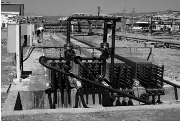
11.9 Concrete storage module (PSA-Almeria) before installation of insulation.
