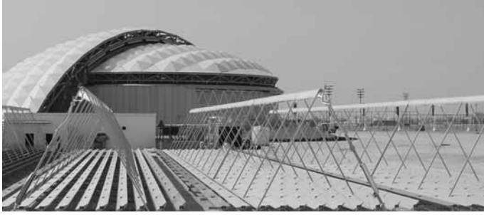
19.8 Fresnel collector field by Industrial Solar GmbH in front of showcase football stadium in Doha, Qatar.
