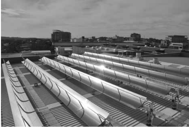
19.2 Parabolic troughs for a solar cooling system in Newcastle, Australia (source: NEP Solar AG).
