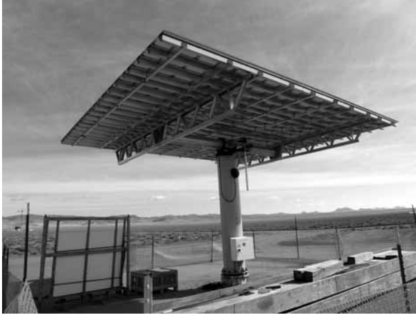
8.10 SolarReserve demonstration heliostat on Crescent Dunes site, November 17, 2011, 170 m concrete tower completed February 9, 2012, awaiting addition of cylindrical receiver (SolarReserve, with permission).
