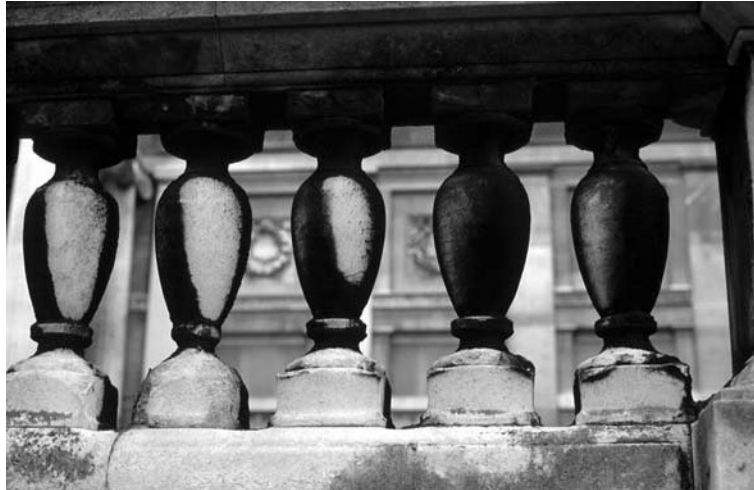
Plate 6.4 Weathered balustrade on the Ashmolean Museum, Oxford, England. The balustrade has now been cleaned. (Photograph by Heather A. Viles)
