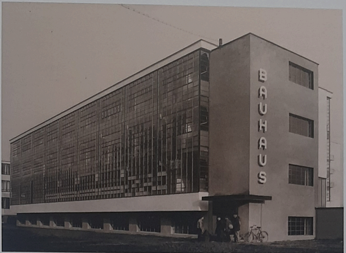
Anonymous: Walter Gropius's Bauhaus building in Dessau. View of the Bauhaus building from the southwest, workshop wing, 1925/26
