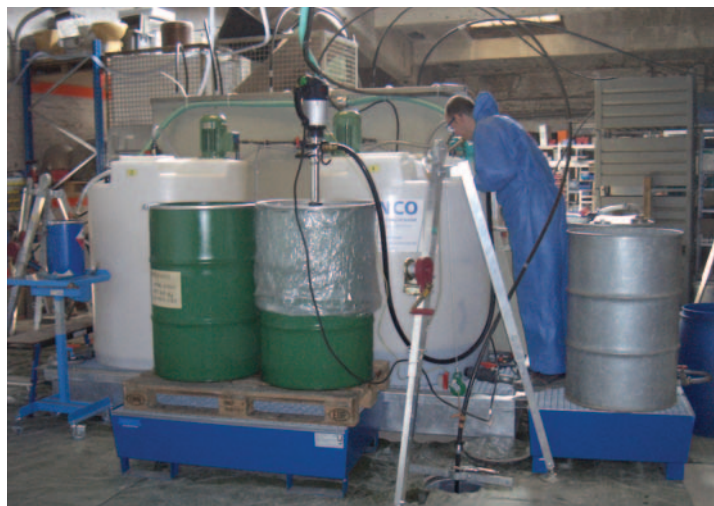
FIGURE 4 Mixing station where the iron particles in the slurry are resuspended before injection. © ALENCO GMBH, GERMANY
