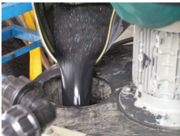
FIGURE 3 nZVI slurry being poured into a well. © AQUATEST, CZECH REPUBLIC
