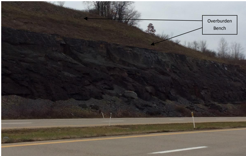
Figure 8.6.1-1 – Example of an Overburden Bench
