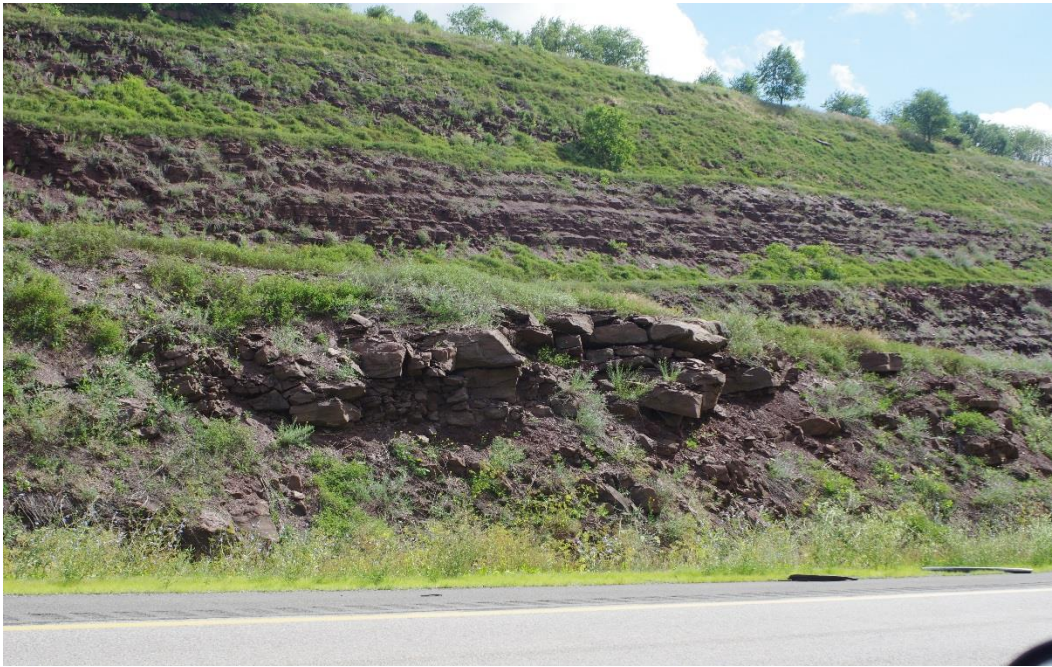
Figure 8.6.2-1 – Example of a Geotechnical Bench
