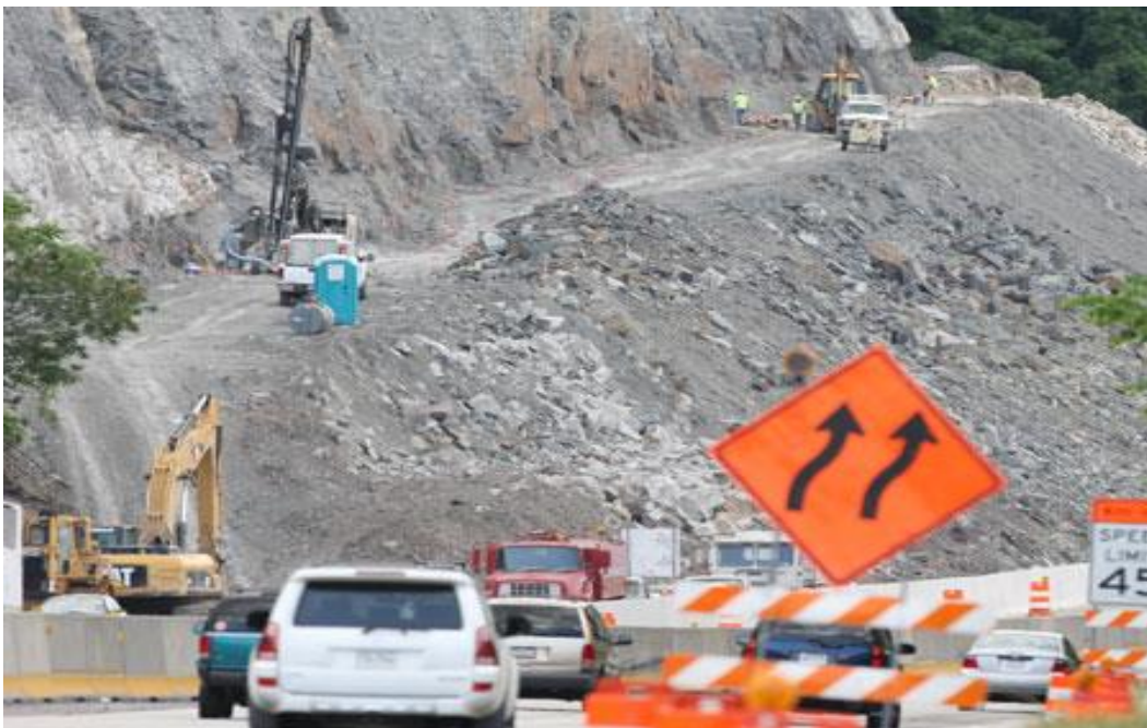
Figure 8.6.3-1 – Example of a Construction Bench
