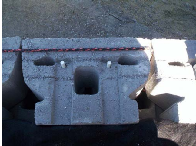
Figure 15-(KeySystem I)-1 Keystone KeySystem I block with fiberglass alignment pins.
