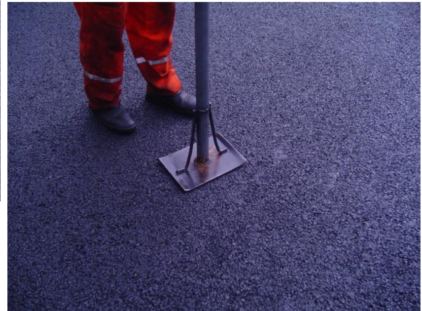
Gap-Graded – camada acabada
