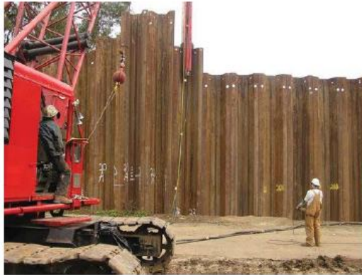
Figure 21.31 Bored piles and sheet pile cantilever walls. (d: Courtesy of Associated Pacific Constructors, Inc.)
