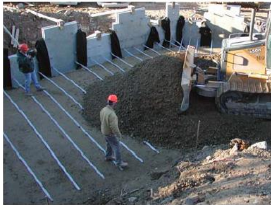
Figure 21.24 MSE wall. (Courtesy of The Reinforced Earth Company.)
