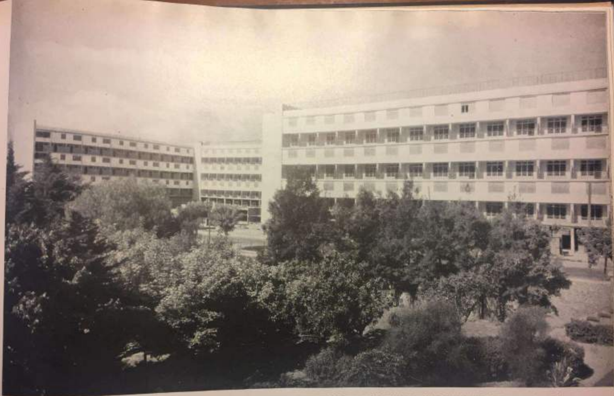
THE RELATION BETWEEN OPEN SPACES AND BUILDINGS. This housing scheme for low-income families, formed by 211 apartments (five-room duplex type), is adapted to the climate of Barcelona (Spain). These apartment units with their community services — branch public library, club rooms, swimming pool, cooperative stores, kindergarden, and public school — form a small neighborhood unit. The widely spaced wings of these blocks and the semienclosed open space between them are reminiscent of the traditional Mediterranean patio and to a certain extent reconstruct this element on an urban scale. The relationship between open and built-up spaces is especially important in housing schemes; from it may be derived a great variety of architectural expressions.
