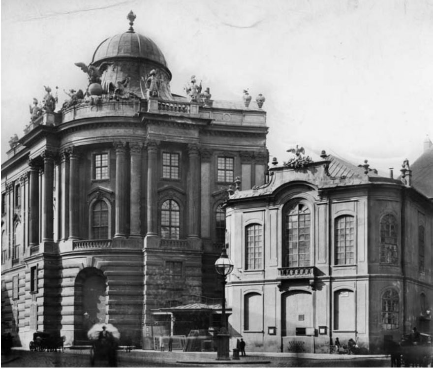
Figure 8.2: A photograph of the Burgtheater (on the right) in 1885, shortly before its demolition
