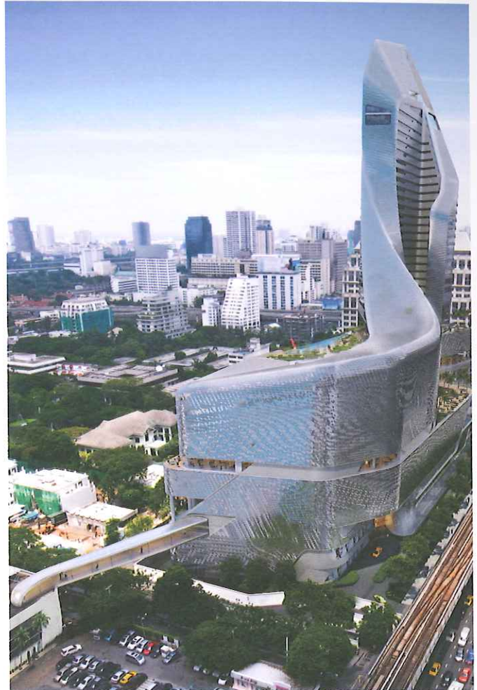
The application of algorithmic design software for the Central Embassy in Bangkok by AL_A allowed a high level of visual complexity across the building's envelope through the interaction of three-dimensional tiles across the large surface area.
