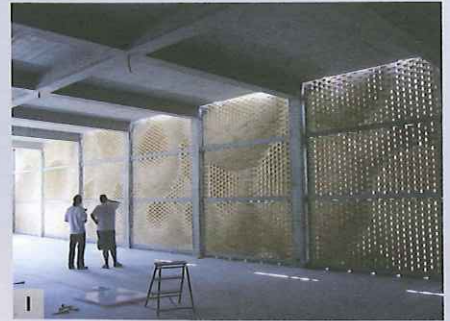
G The wall elements were manufactured as a pilot project in research facilities at ETH Zurich, transported by truck to the construction site, and craned into place.
