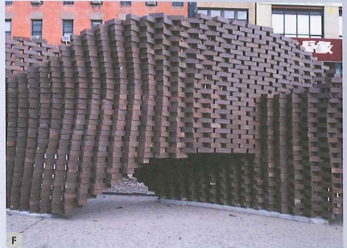
F The digitally designed brick structure is further articulated using a weighted compressing and tensioning of the brick bond. Where the loop "flies," the bond becomes stretched and thus lighter; where it brings loads to the ground it becomes jagged and heavier, thus wider and more stable.
