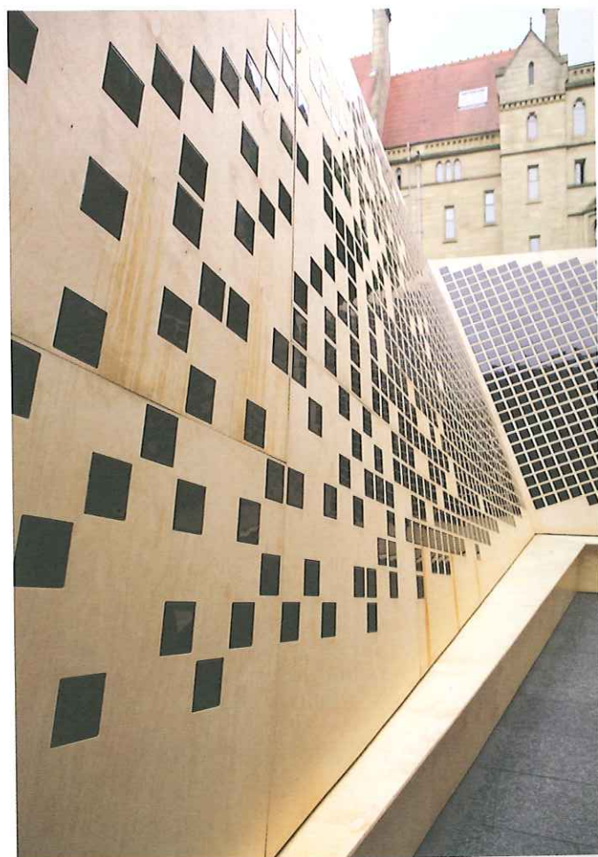
6 The "skin" layers were manufactured oversized, allowing on-site adjustments to accommodate the geometries of the synclastic, curved surface. Manual construction skills allowed adjustment to take place in order to resolve problems found on site.
