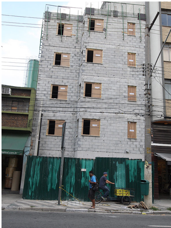
Picture 3.20. Construction Site at São Caetano Street, May 2016
