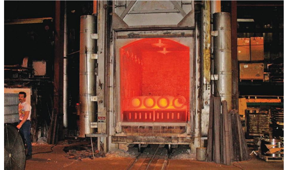
Fig. 1. Typical gas-fired furnace with low-NO x burners at a commercial heat treater
