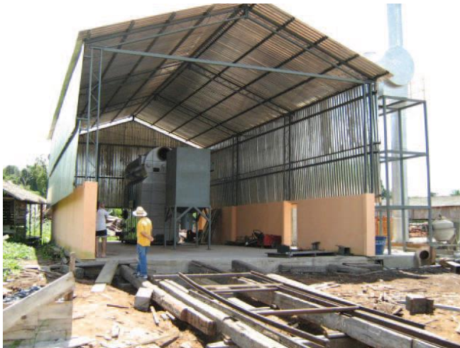
3. Installation of the equipment
