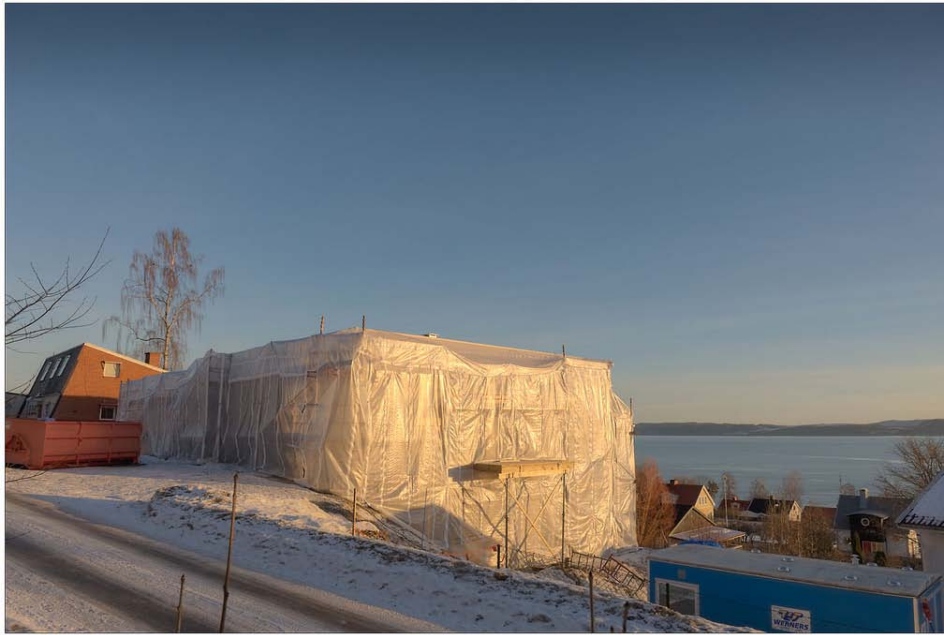
Figure 1. Private residence project in construction with weather protection to avoid climate or moisture related building defects during the building process. (Photo: Augustinius J., 2011)
