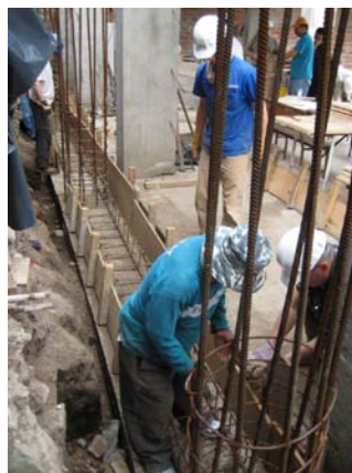
Figure 3: Grade Beam
