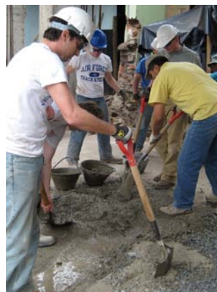
Figure 6: Mixing Concrete
