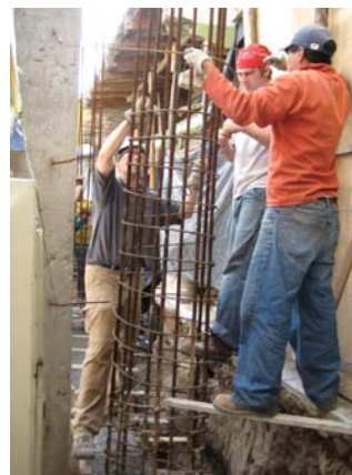
Figure 4: Column Rebar
