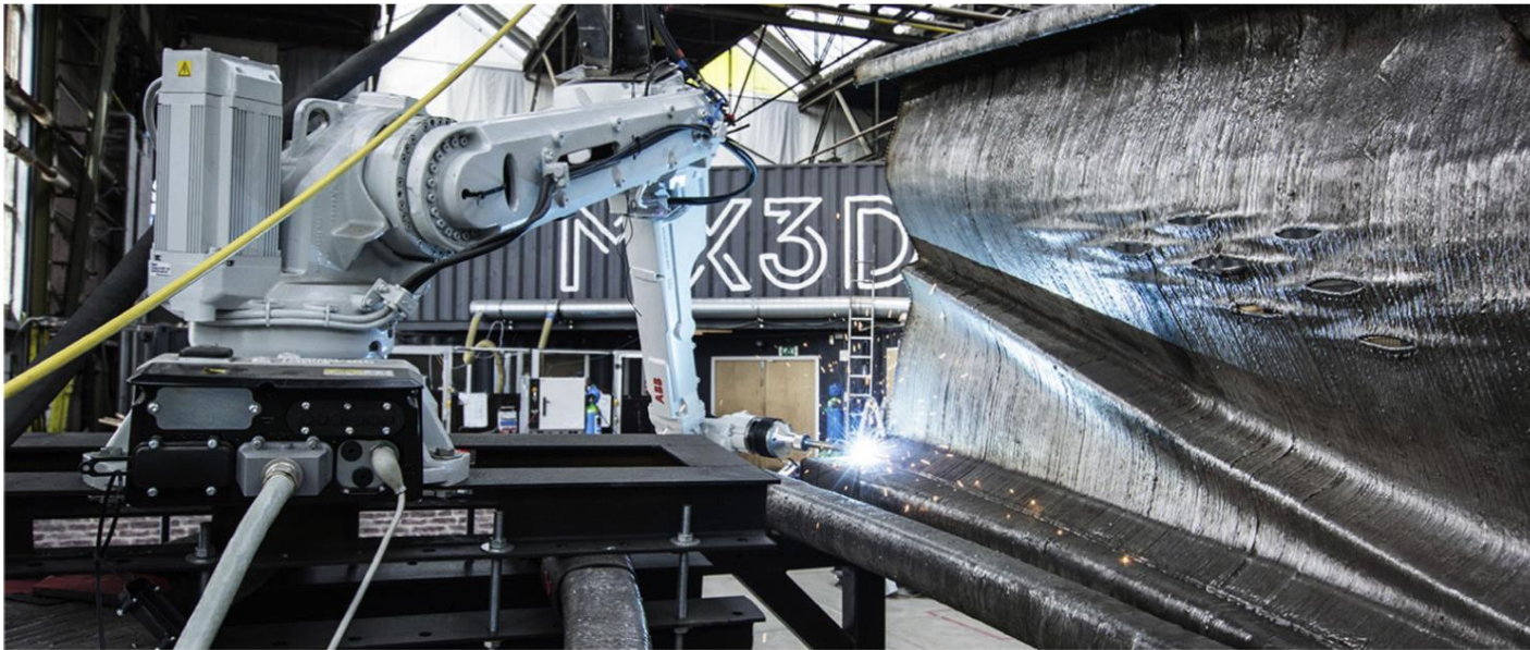
Fig. 4. Metal bridge part manufactured with the MX3D printer [103].
