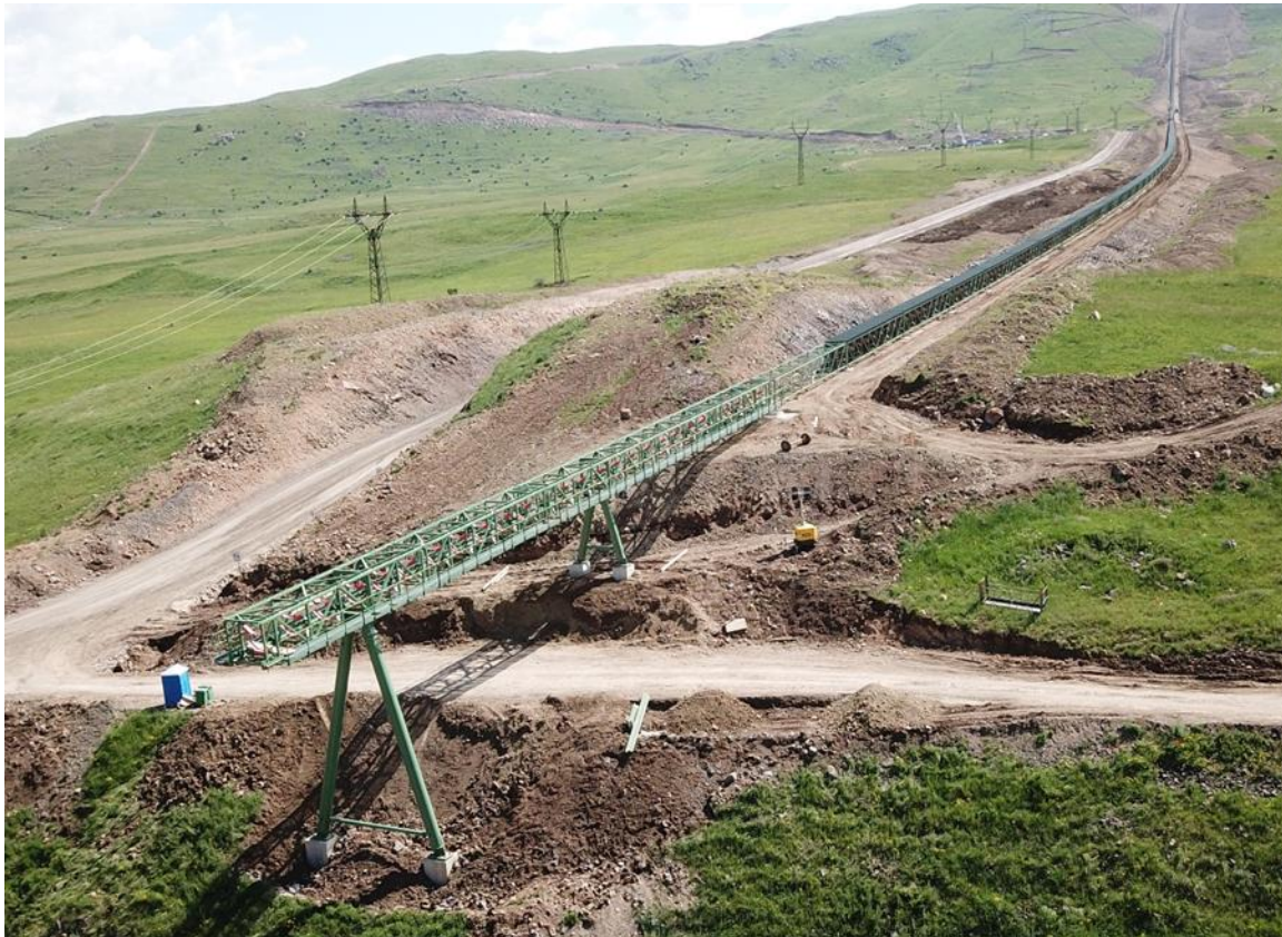
Figure 4-5: Construction of Overland Conveyor and Power Distribution
