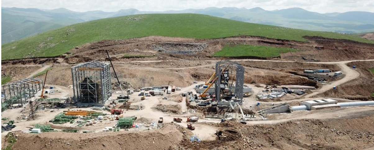
Figure 4-4: Construction at PL12 (Crusher)
