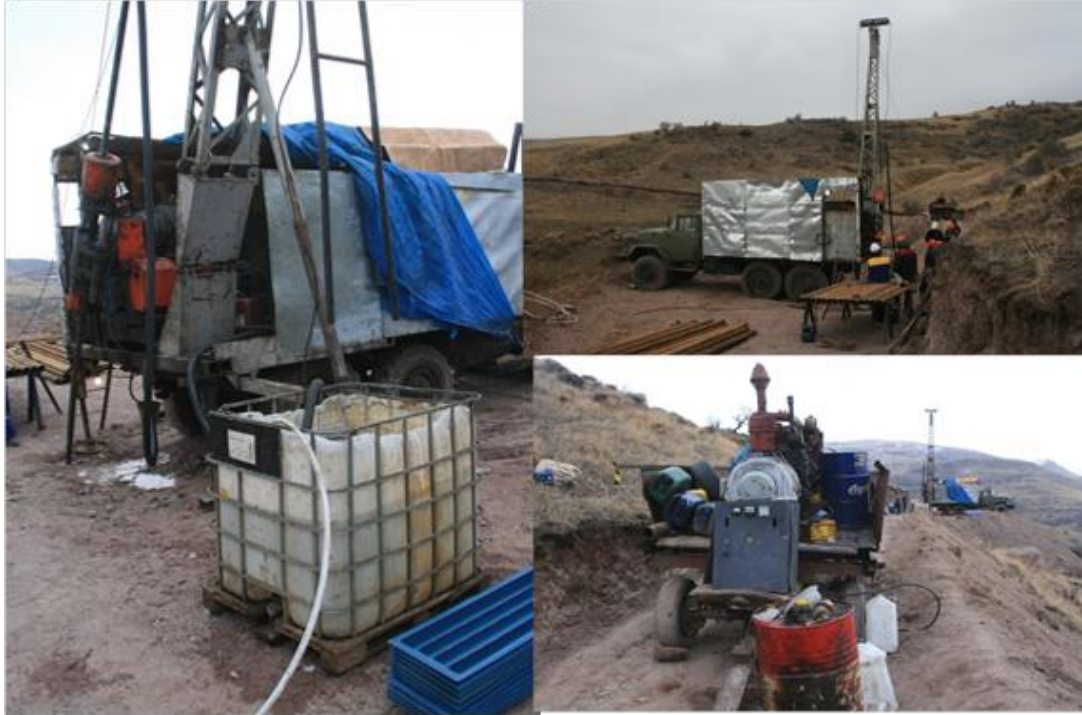
Figure 10-2: Drilling Operations Amulsar Project
