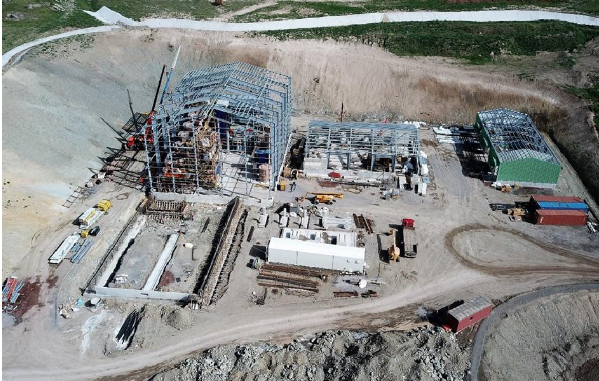
Figure 4-6: Construction of ADR Plant and Associated Facilities
