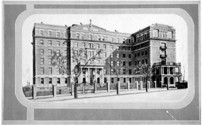
Figure 2: High-tech departments like surgery were subtly visible in the façade of Hôpital Notre-Dame. A. Adams. Source: Courtesy of the author
