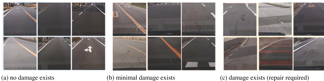
Fig. 10. Dataset labeled by expert road managers to train the CNN model [27].
