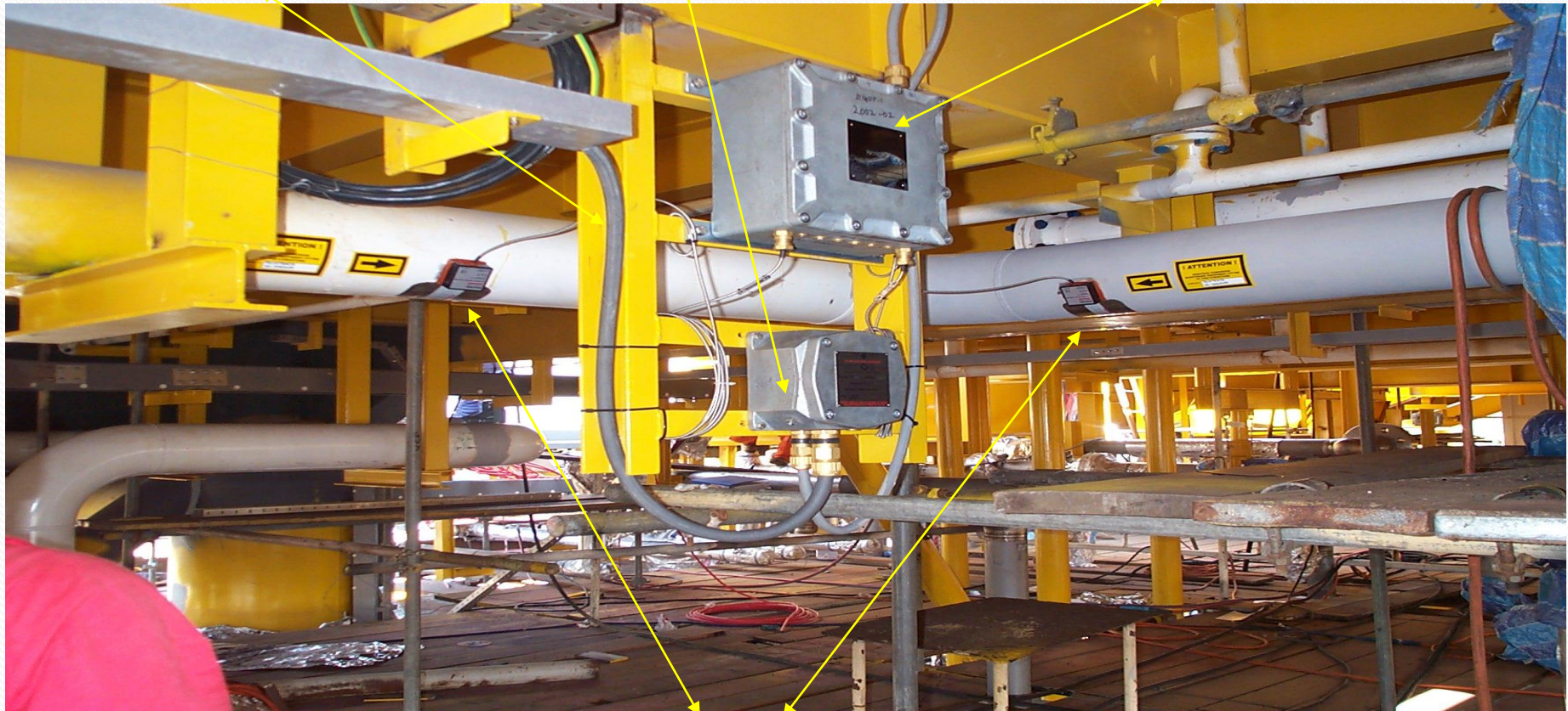
A RIGHTRAX Installation site showing Installed Sensors Prior to The Customers Paint and Insulation being applied to the piping system
