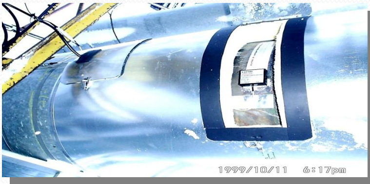
M1 sensors Fitted on Pipelines prior to insulation be reinstated
