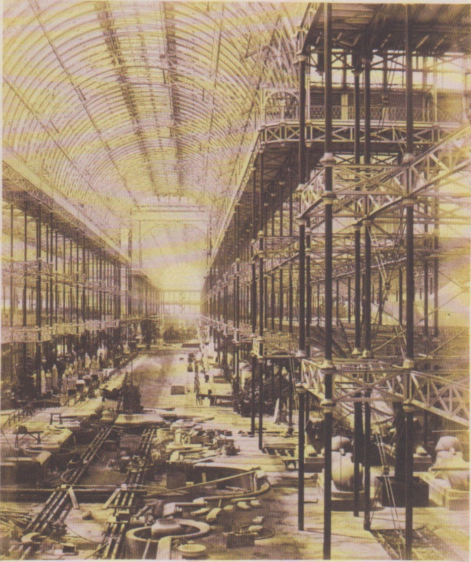
127. The Nave from the North end—Commencement of Monti's Fountain.
