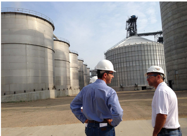
Figure 18.4. The Tharaldson Ethanol plant in North Dakota uses municipal wastewater and returns about 25% of the volume at drinking water quality to the city of Fargo ( www.tharaldsonethanol.com ).
