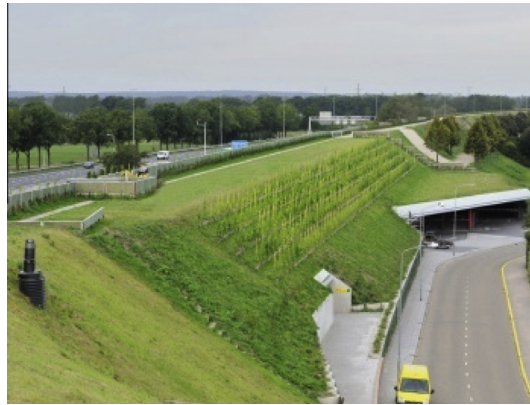
Fig. 3. The parking garage of the CineMec in Ede is built into the noise barrier for the A12 motorway in the Netherlands. Source: http://zakelijk.cinemec.nl/content/4194/bereikbaarheid.html , accessed in June 2014.
