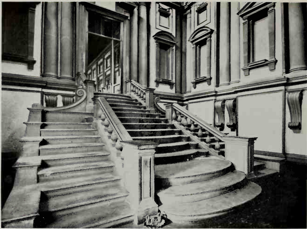
18a. Laurentian Library. Vestibule stairway.
