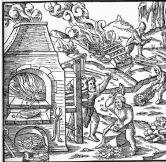
A—WOOD. B—BRICKS. C—PAN. D—FURNACE. E—CRUCIBLE. F—PIPE. G—DIPPING-POT.
