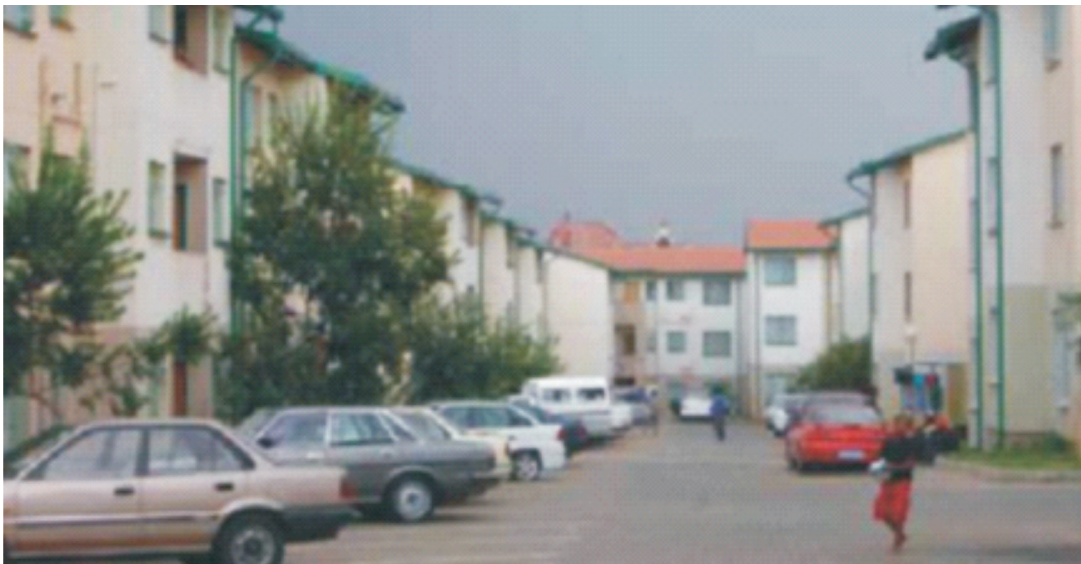
Figure 2 — Newtown Urban Village: COPE's 351-unit Social Housing Development in the Johannesburg CBD.
