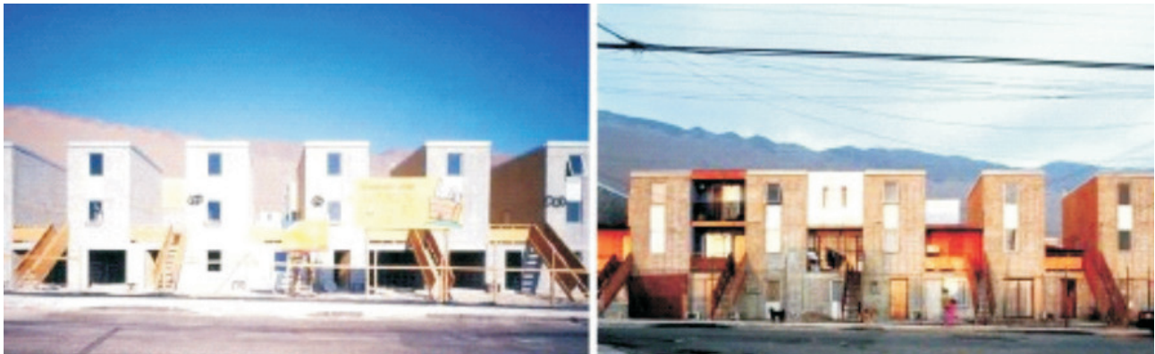
Figure 10 — Example of architecture designed to allow for an organized expansion of the living area. The Quinta Monroy, as built (left) and after intervention by users (right). Source: Elemental Chile ( www.elementalchile.cl )
