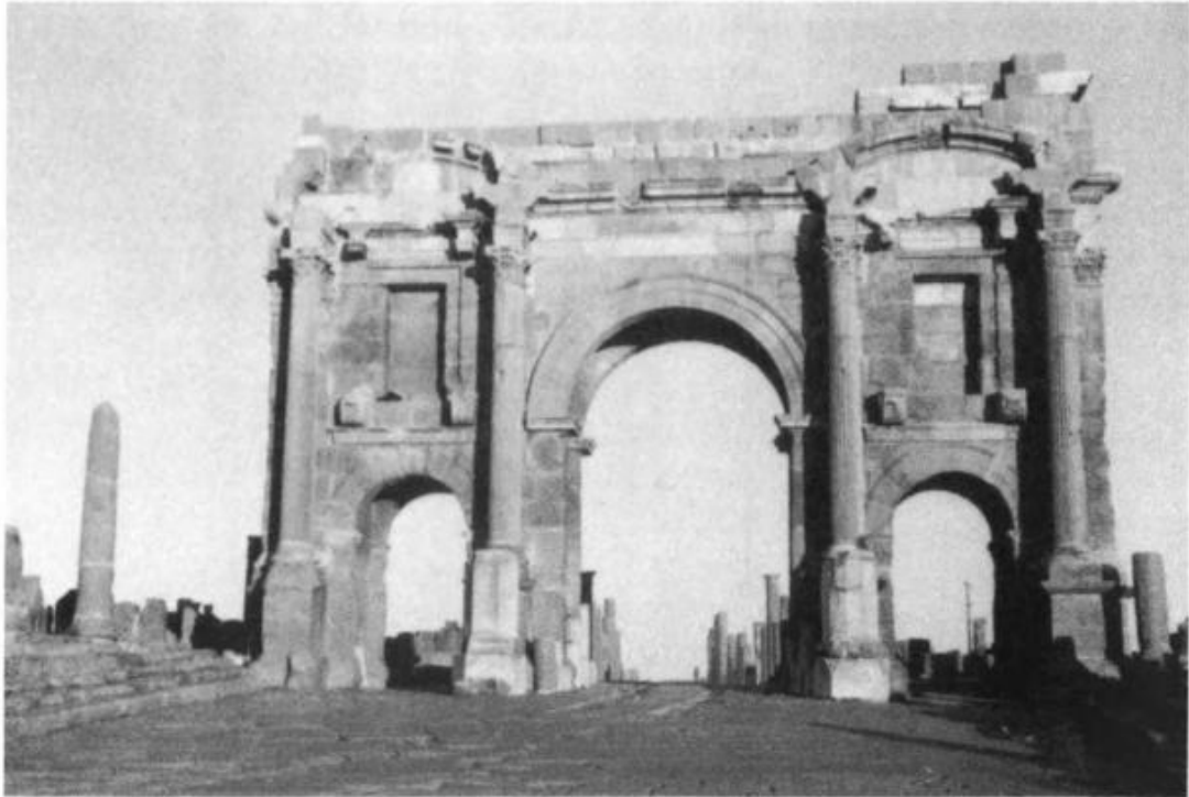
Arch of Trajan, Timgad: travellers from Lambaesis arrived by this road. The grooves worn by wheeled traffic are clearly visible
