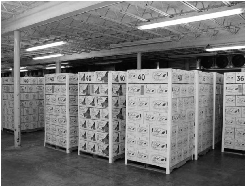
FIGURE 17.30 Room cooling. Refrigerated air is circulated throughout the room using the evaporator fans mounted near the ceiling in the back of the room. Cooling is only through passive convection. In this case, the small area for carton ventilation will result in very slow cooling times.
