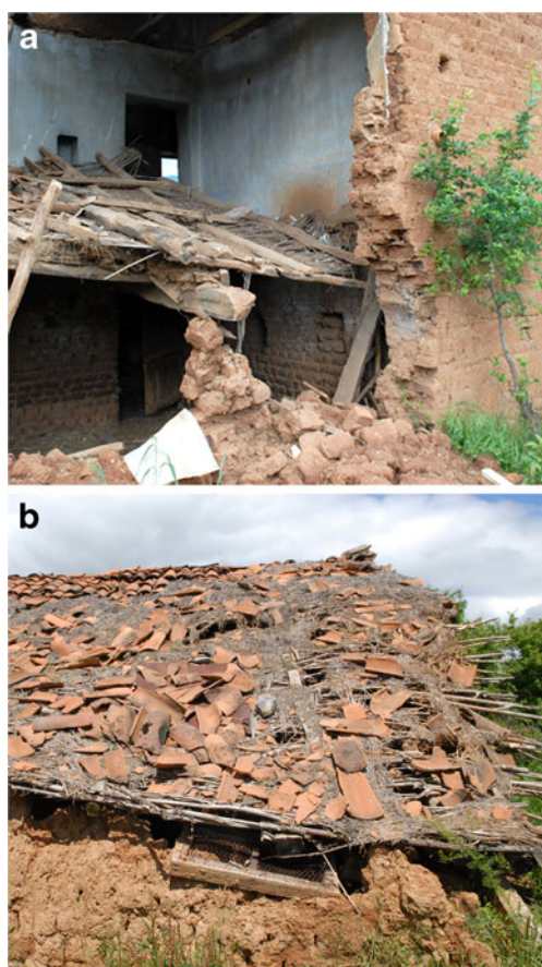
Fig. 3 Examples of construction tradition in Kranionas. a Typical two-storied mud house with animal shelter at the ground floor and human habitation space at the upper floor. b Roof made of wooden beams covered by reeds and small branches covered by commercial roof tiles
