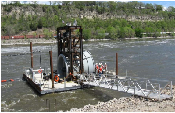
Fig. 8. A 100-kW Nameplate Capacity hydro-kinetic unit. This unit is located at the U.S. Army Corps of Engineers Lock and Dam No. 2 in Hastings, Minnesota. (Used with permission of Hydro Green Energy, LLC).
