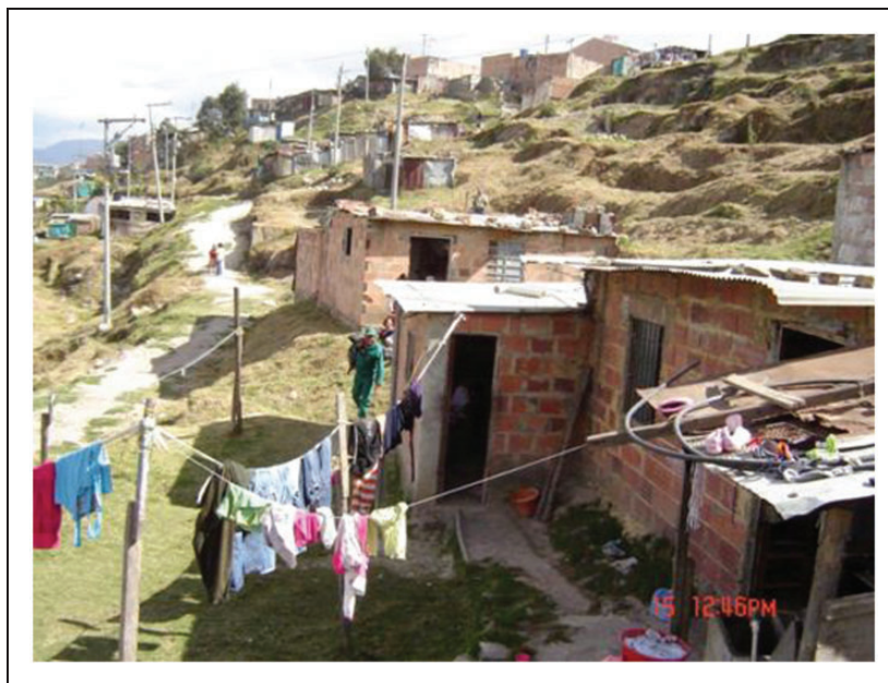
Figure 4. Original settlers' houses in the Altos de Estancia high risk zone. The owners, settled in the zone since the 1990s, needed to regularise the family's land titles before admittance to the resettlement programme, and were negotiating for two new houses through the resettlement programme to accommodate all family members.
